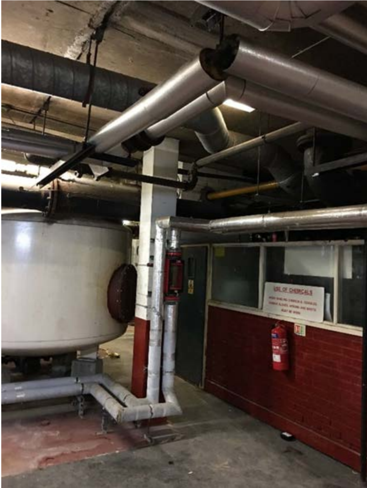
Fig 4.1.5 – The photo above was taken with the basement area.
