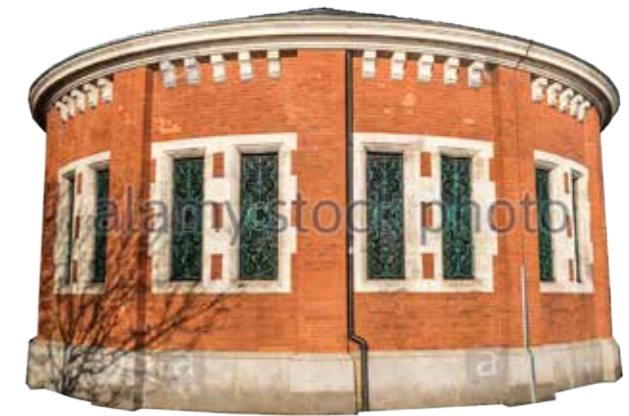
4. Grade II listed Rotherhithe Ventilation Shaft rotunda
