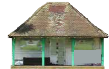
5. Existing bowling green pavilion to be renovated as sports store
