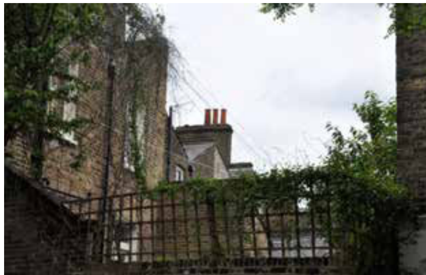
Glimpsed view of butterfly roofs from Zealand Road.
