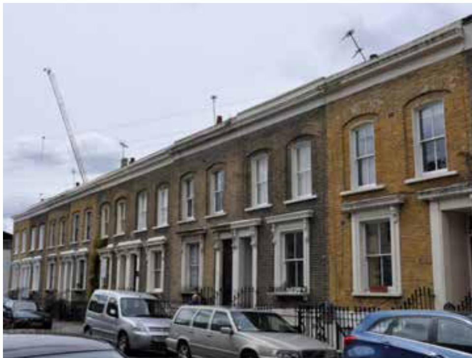
Two storey houses, with basements, along Ellesmere Road.
