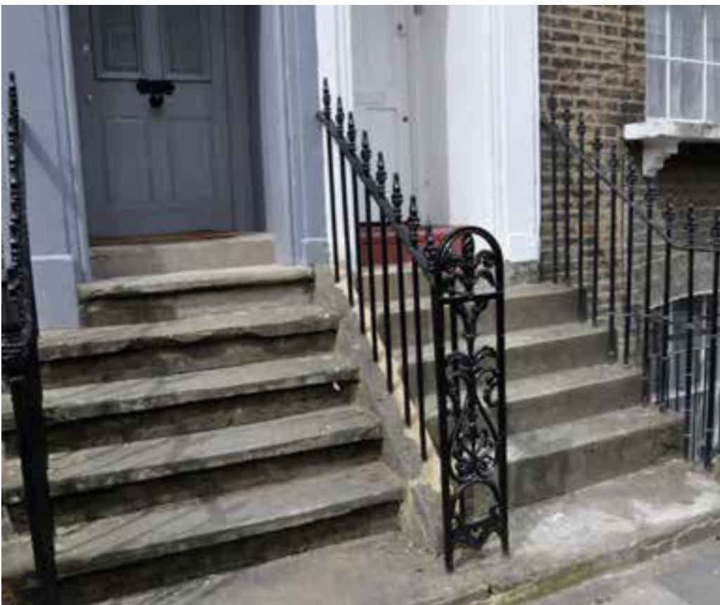
Below: Original wrought ironwork boot-scraper situated between two houses on Driffield Road. This design feature is also found on Grove Road. Also note, the loss of stone nosings to the modern steps on the right.
