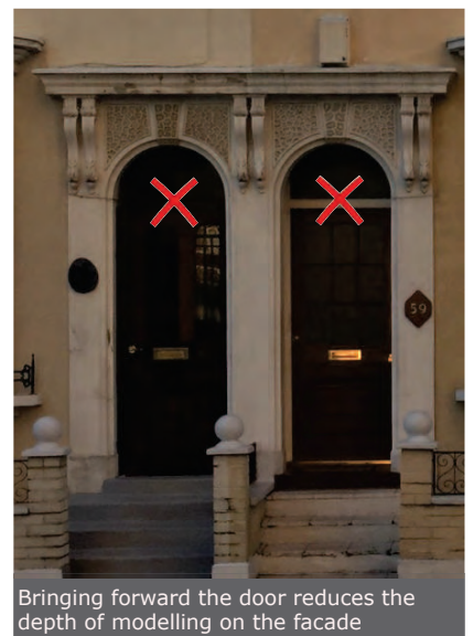
Bringing forward the door reduces the depth of modelling on the facade
