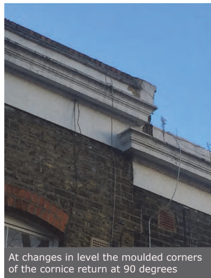
All render requires regular maintenance and redecoration; cracks lead to decay
