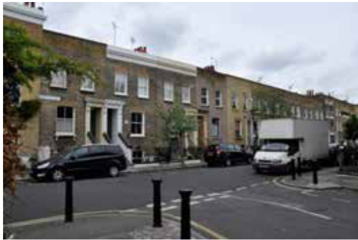
View of Chisenhale Road from top of Zealand Road.
