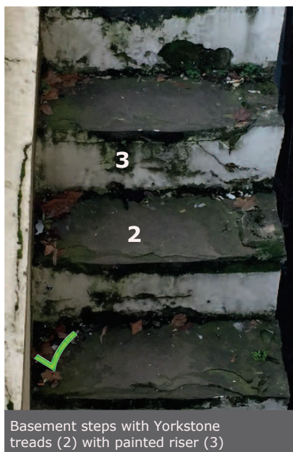
Yorkstone projecting nosing (1), tread (2) and riser (3)
