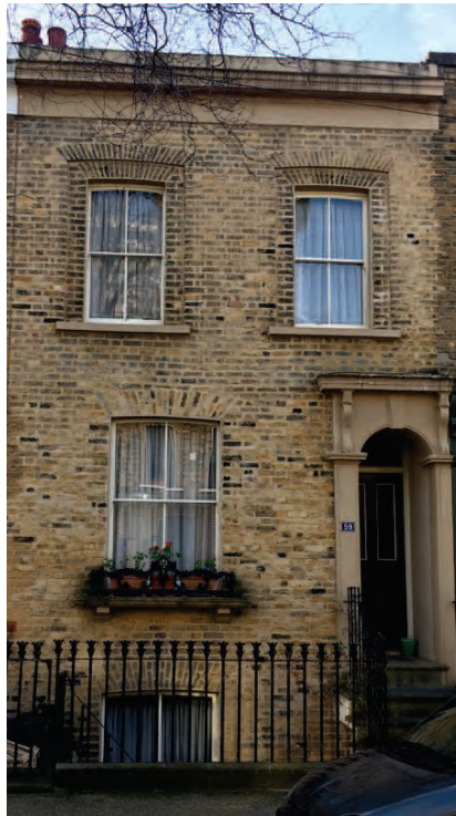
Property with original features intact
