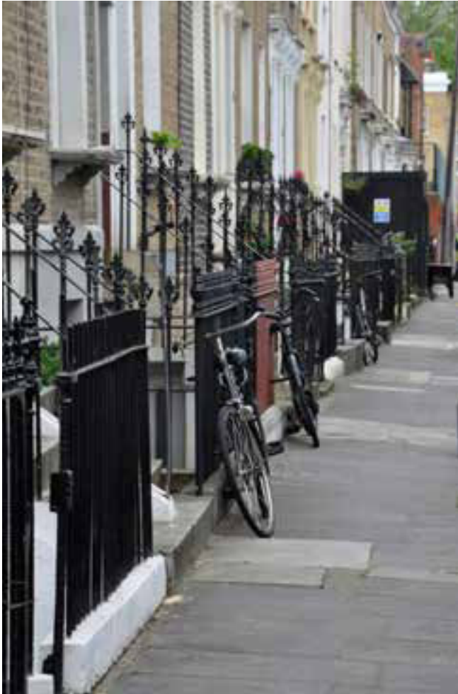
Opposite: Original railings along the west side of Zealand Road.
