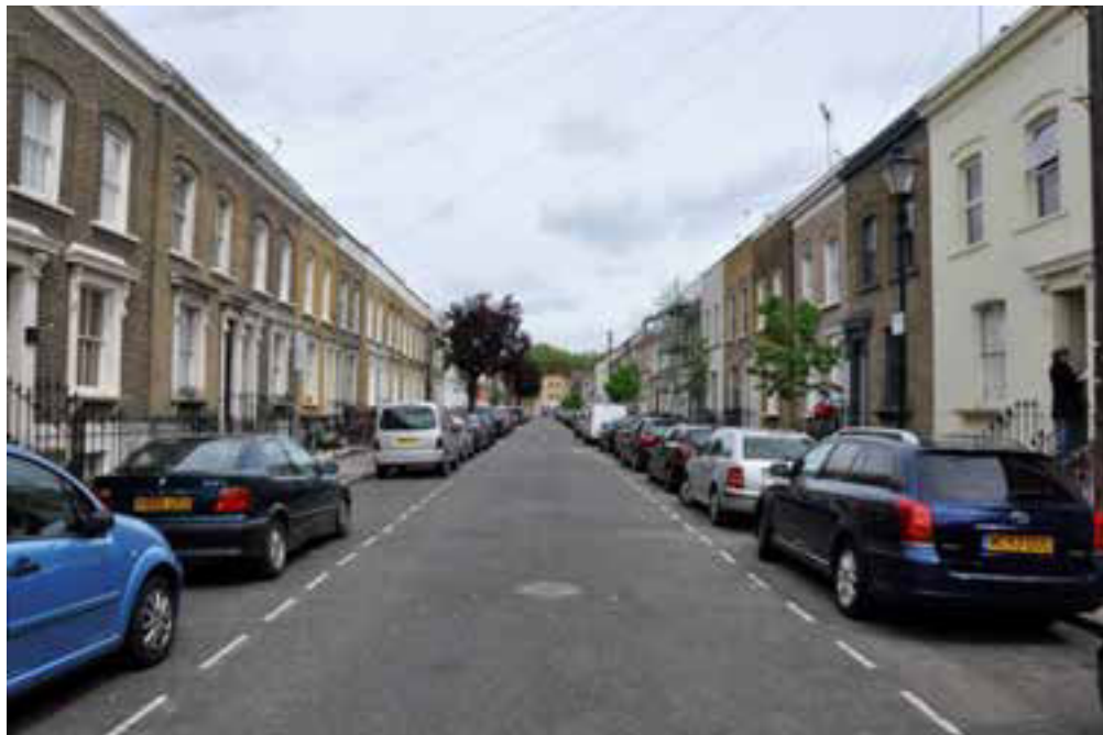
View looking up Ellesmere Road from Roman Road. The continuous line of the roof and of decorative features such as the cornice gives the terrace a rhythm and symmetry.
