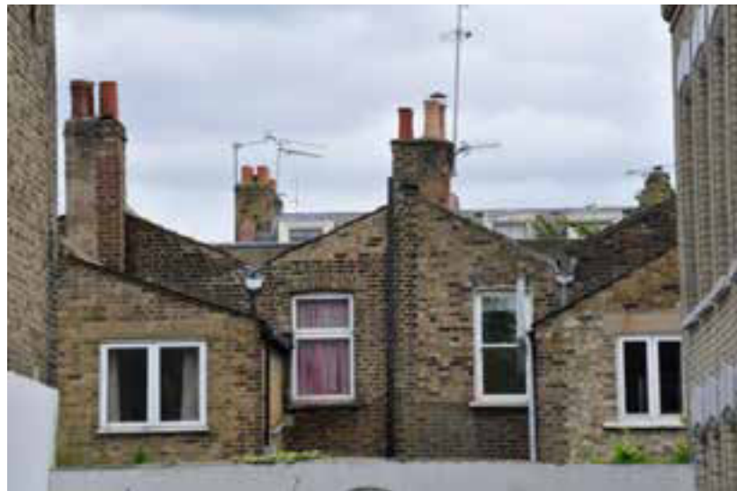
The rear elevation of the butterfly roofs of properties on Kenilworth Road, as seen from Grove Road. Note also the pairs of chimney stacks located along the party walls.
