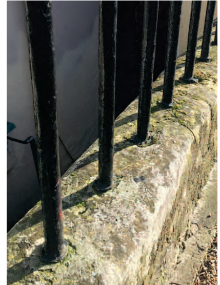
Bars lead caulked into stone base
