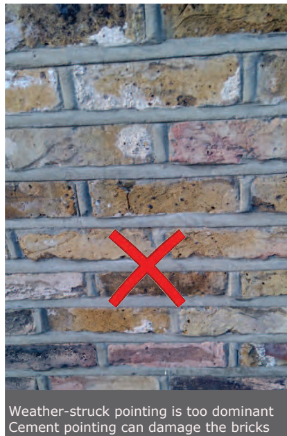
Re-pointing should be in lime mortar set behind the face of the bricks
