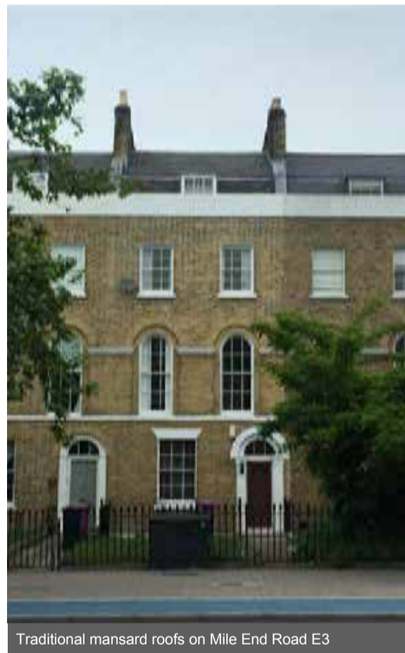
Traditional mansard roofs on the corner of Mile End Road and Tredegar Square E3
