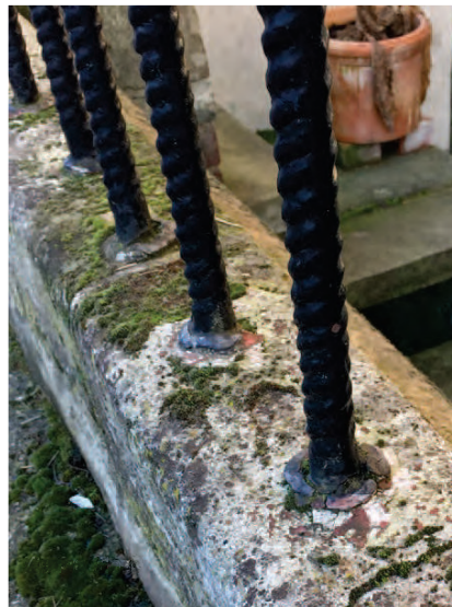
Bars lead caulked into stone base
