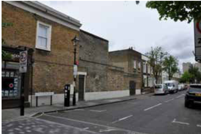
View from bottom of Kenilworth Road: side elevations of houses clearly visible.
