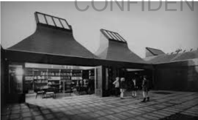
Bromley Hall School, 1969: folding doors open up the library to its adjacent court.
