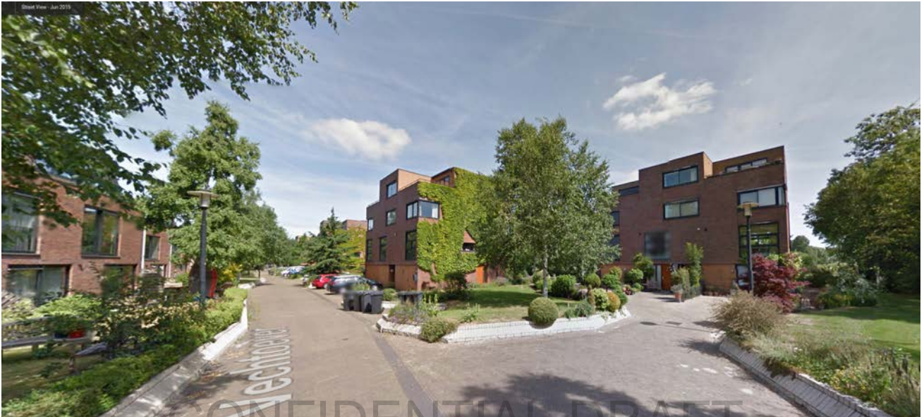
Kop van Zuilen, Utrecht Buildings in the public green space, on street parkin
