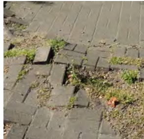
Blockwork paving appropriate to remove - Silvocea Way
