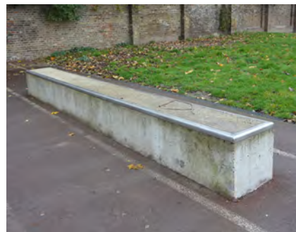
Cast-in metal edgings can prepare street furniture for skaters; Normand Park, London
