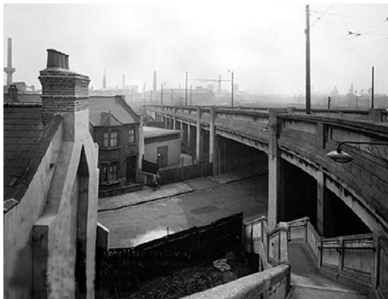
Historic photograph of the viaduct (1939) Having been designed to accommodate the large volume of heavy traffic that serviced the Royal Docks, the viaduct has a generosity and structural significance that could be exploited.
