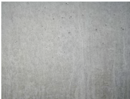
FAIRFACED CONCRETE Concrete channel benches - vertical surfaces
