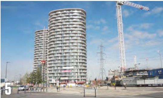
Tidal Basin Road towers, residential and hotel - under construction
