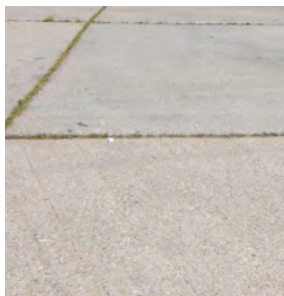
Insitu Concrete - North of A13
