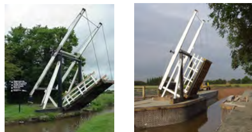
An example of a Bascule bridge crossing similar to that proposed at of Cody Dock - this project will replace the existing dock crossing, and has planning approval, allowing the dock to be used for moorings.
