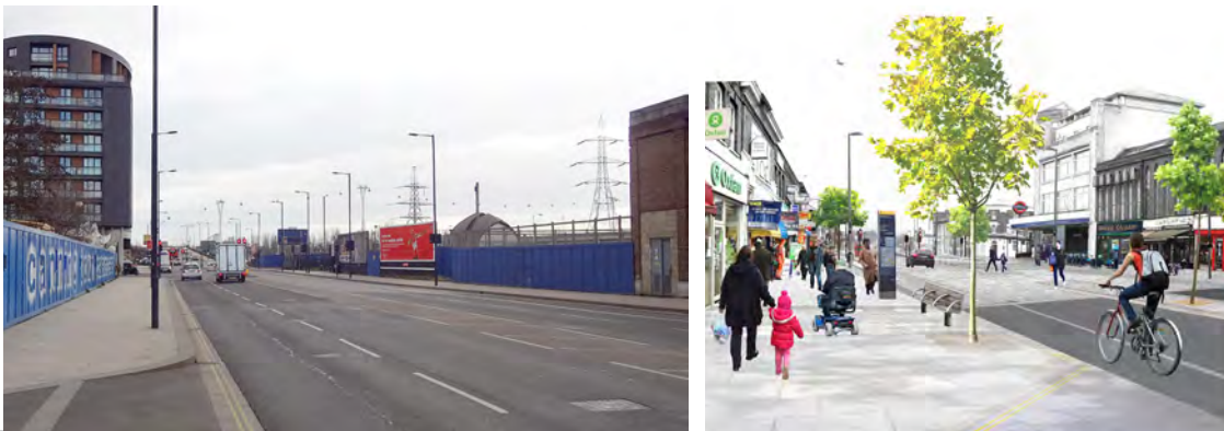
Develop a public realm and planting proposal which aims to both meet TfL Streetscape guidance and act to create a sense of place
