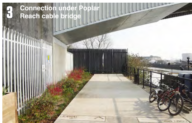
Poplar Reach cable bridge: a structure designed to allow a pedestrian path beneath it but which has formed an obstruction for 20 years.
