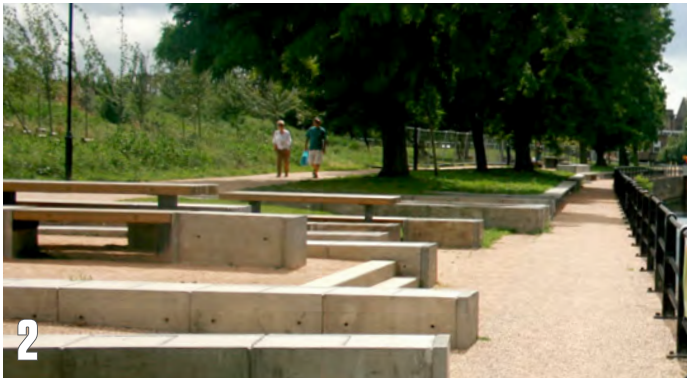
Precast concrete channels in use at Three Mills Green
