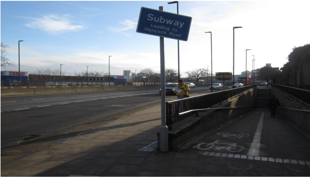
View looking south along A12 Trunk Road
