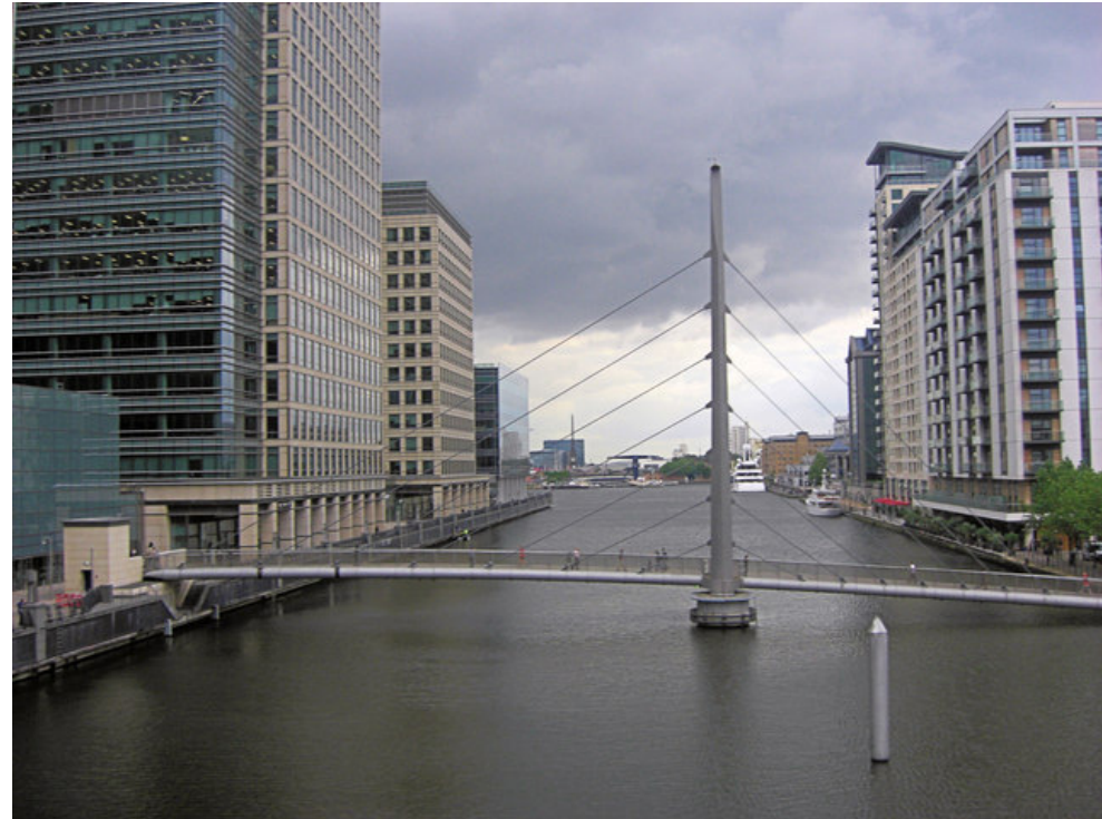
The existing footbridge between South Quay and Canary Wharf
