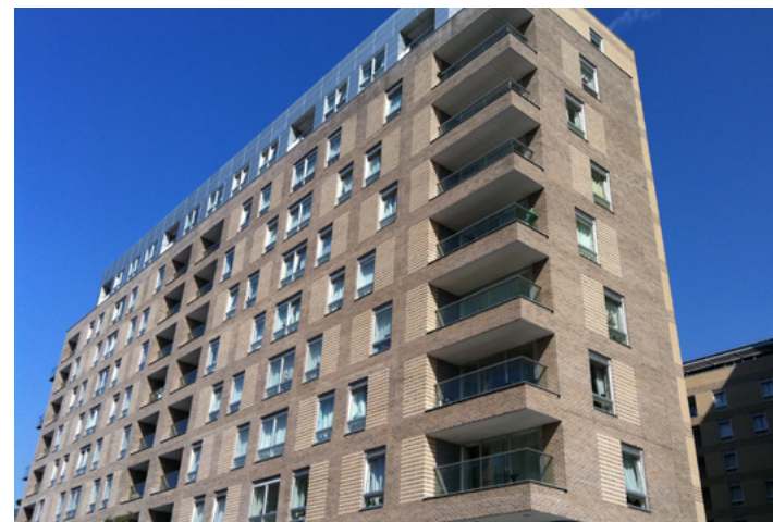
Baltimore Wharf development near Crossharbour DLR Station
