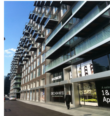
Baltimore Wharf development near Crossharbour DLR station
