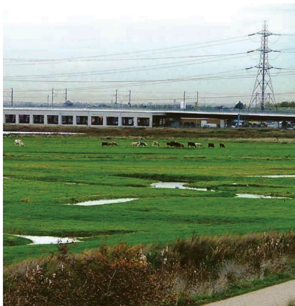
High Speed One (CTRL) crossing Rainham Marshes on piled raft
