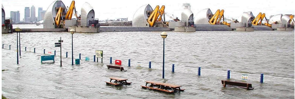
Surge tide event at the Thames Barrier
