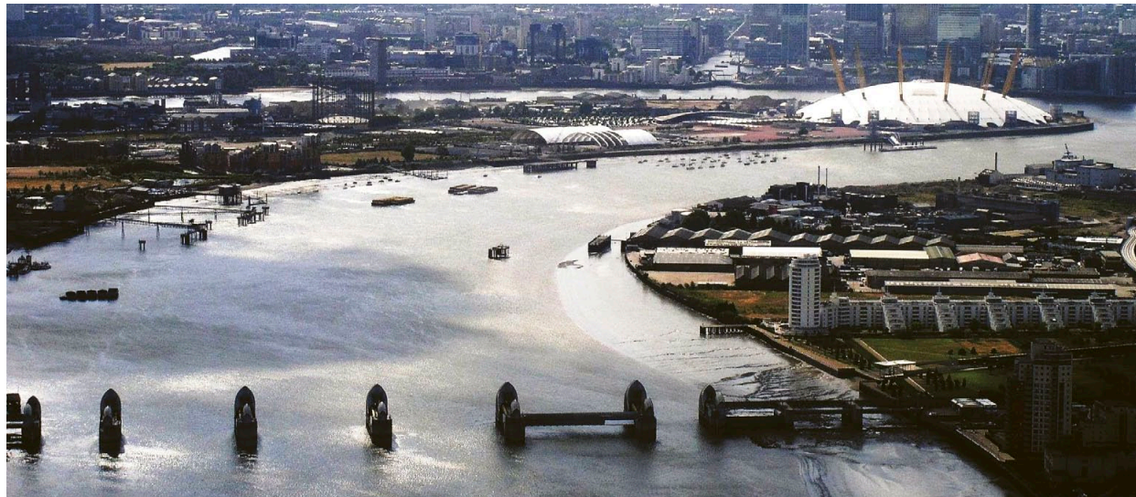
The Thames Barrier has remained a constant feature in the rapidly changing urban landscape over the past 25 years
