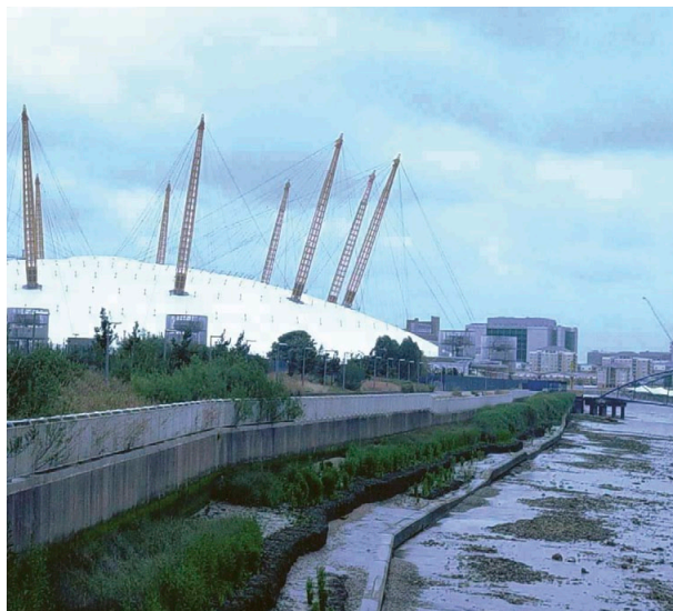
Terraces at the O 2 – cheaper to build, subsequently increased value of the land and enhanced local ecology
