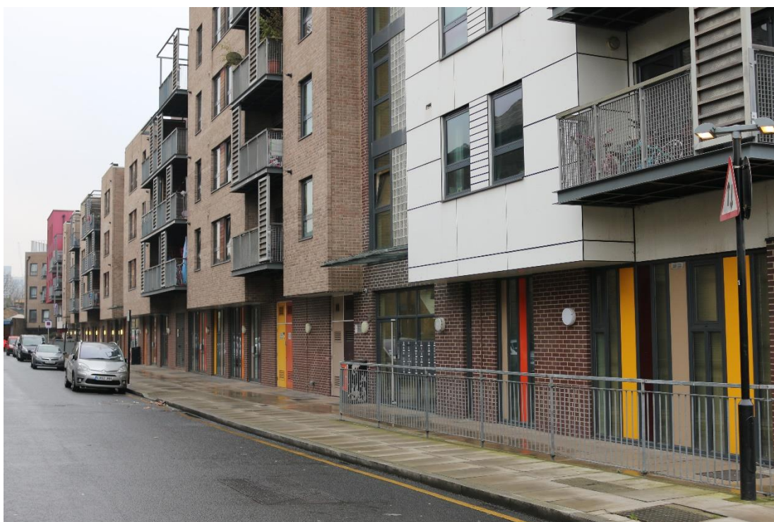
Figure 4.18 ACME-run artist studios on the ground floor of affordable housing units on Leven Road
