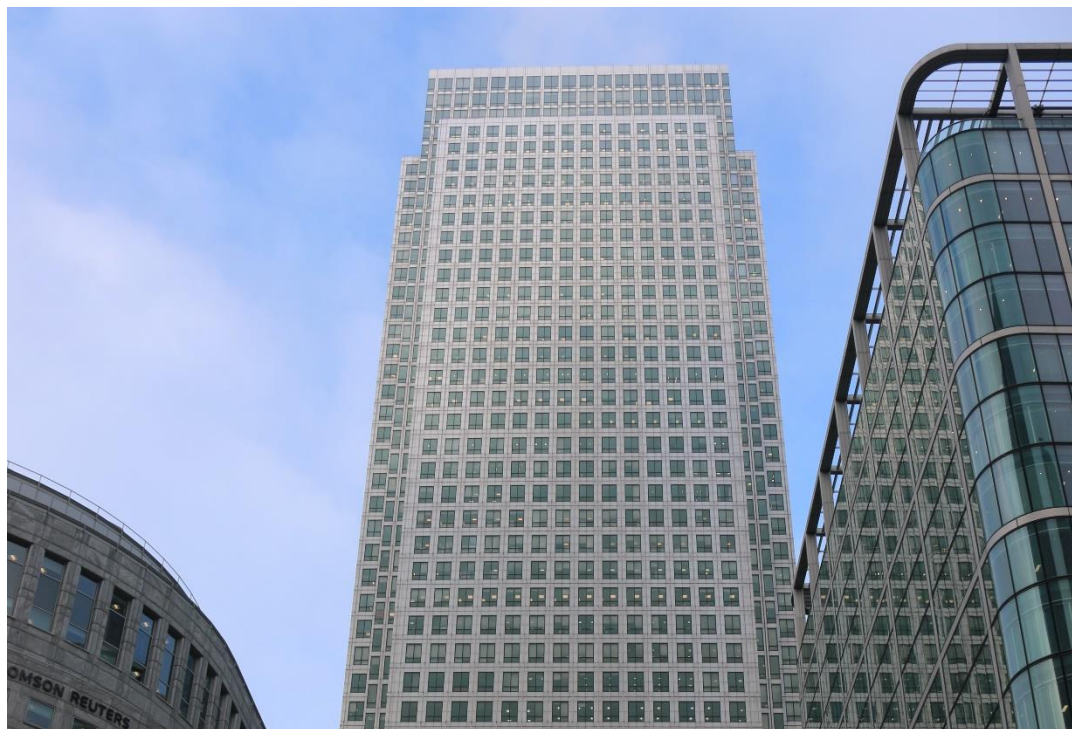
Figure 4.17 Co-working spaces and IAC spaces are offered on particular floors in One Canada Square
