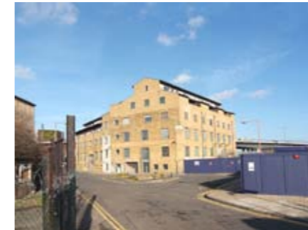
Warehouse in Leamouth
