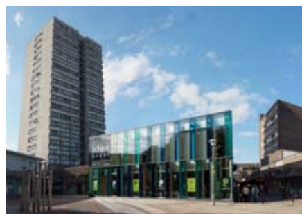
Idea Store on East India Dock Road
