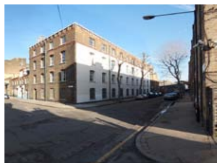
Historic warehouses in Fish Island
