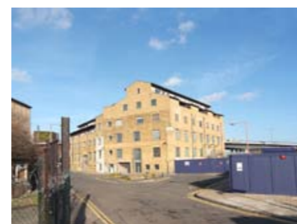
Warehouse in Leamouth
