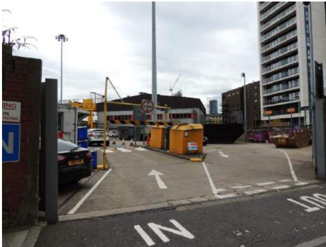
Photo 1: Showing Access to HWRC
