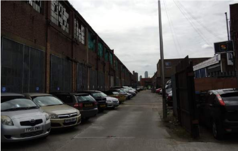
Photo 9: Showing disused warehouse & occupied units to right
