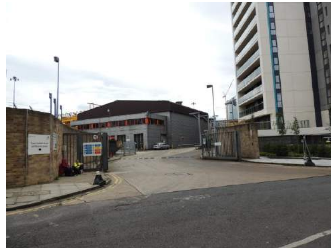
Photo 2: Showing access to WTS & Wharf
