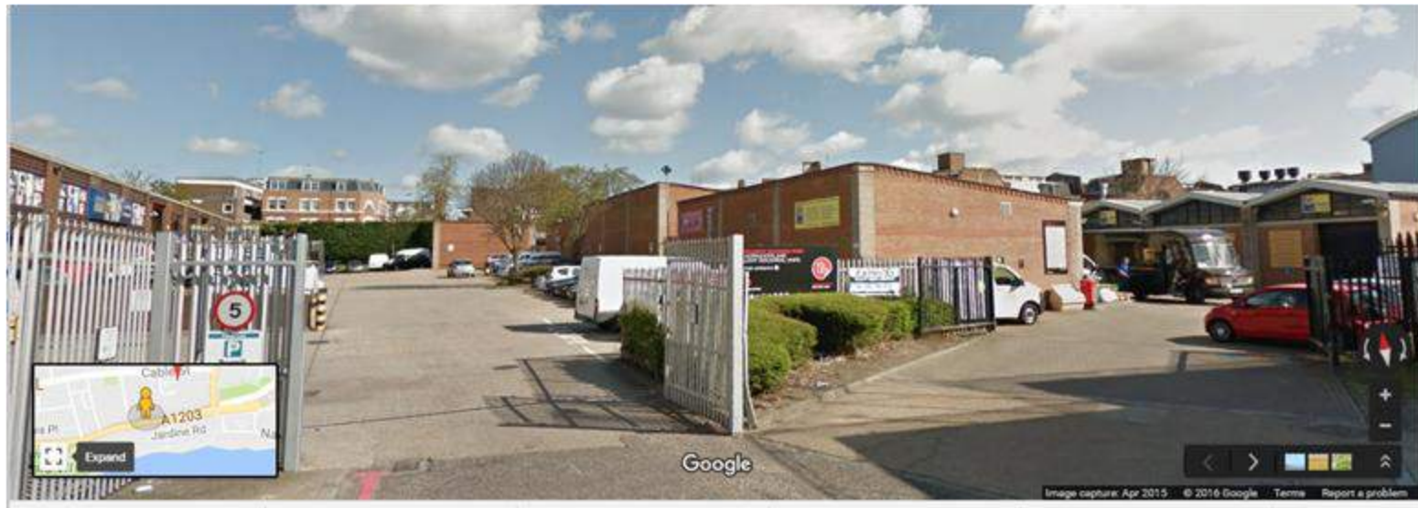
Photo 6: Access & egress from public highway to two estates
