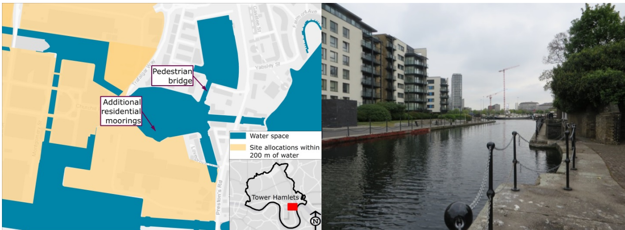
Blackwall Basin and Poplar Dock proposed infrastructure. Interface between Blackwall Basin and Poplar Dock.
