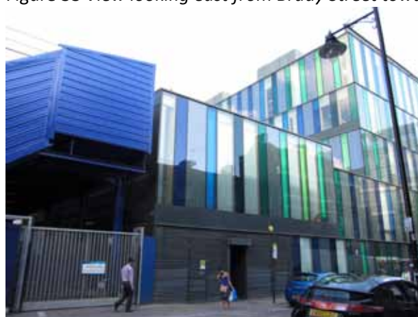
Current view looking east from Brady Street towards back of IDEA store
