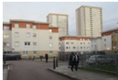
C. The post-war British Street Estate, developed between 1969-1976, contains 500 dwellings. It comprises two 22-storey tower blocks and numerous low-rise block of flats and maisonettes. It was recently refurbished.
