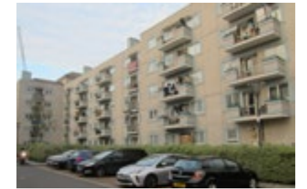
F. Early post-war blocks of 4-6 storeys with a regular grid and projecting balconies. Pitched roofs and other features were added between 1998-2000.
