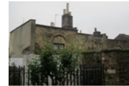
E. The Grade II listed St Paul's Terrace, a 1820 stepped 2-storey terrace of 1-bay houses built of stock brick, giving onto a courtyard below.
