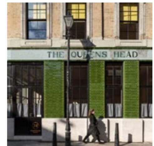
The differentiation in the façade makes the separation between the upper and lower floor uses clear. (photo ©Chris Dyson & Peter Landers Photography)
