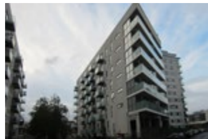
A. Mixed-height linear blocks of up to 10 storeys built in the 2010s, with views facing towards Limehouse Cut.
