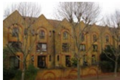
A. Late 20th Century 2-3 storeys-high Sir Thomas More Court built in brick.
