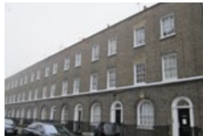
B. Victorian terraces built in the 1840s, within the Albert Gardens Conservation Area. They are of 3 storeys and basements, and have recessed sashes with glazing bars, those of ground floor with semi-circular heads in double recesses.
