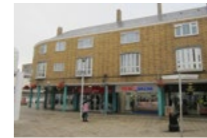
E. Market place with shops on ground floor and maisonettes above built for the 1951 Festival of Britain.
