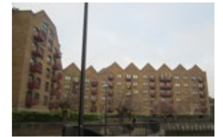
F. Prospect Wharf, a large-scale block of flats built in 1987 on the site of a former warehouse, within the Wapping Wall Conservation Area. 4-5 storeys-high with an elevated ground floor, it is of brick with a concave riverfront and irregular gables.
