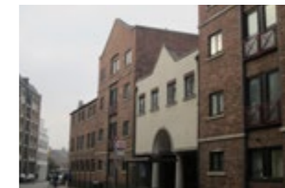
H. Prospect Place, a late 20th Century residential development within the Wapping Wall Conservation Area. The use of brick and the building's wide façades make reference to the area's industrial heritage.
