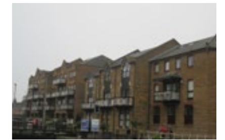
F. Cluster blocks built in 1986 in Goodhart Place, next to Limehouse Basin, with 3-4 storeys, yellow brick and projecting balconies.
