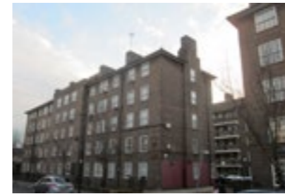
D. 5-storey brick housing blocks from 1929 with a Neo-Georgian façade to the front and utilitarian deck-access at the back.
