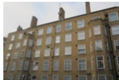
C. Post-war 5-storey housing block on Prusom Street, of yellow brick with bay windows.
