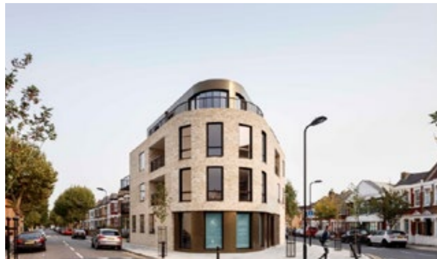
Moore House London (Hackney) HYLO Architects & Matt White architects
