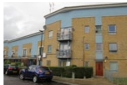
C. 2000s housing development of 2-3 storeys, folded linear blocks for mixed-tenure of approximately 118 units.
