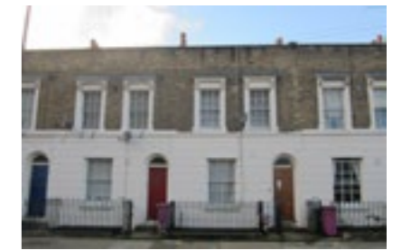
F. Uniform residential terraces with stuccoed lower storey and decorated with stucco mouldings built in 1829-1843, part of York Square Conservation Area.
