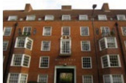
B. Mulberry House, completed in 1936 as part of a slum clearance programme. Part of the Bethnal Green Gardens Conservation Area, the building is Neo-Georgian with 3-storey canted bay windows and brick.
