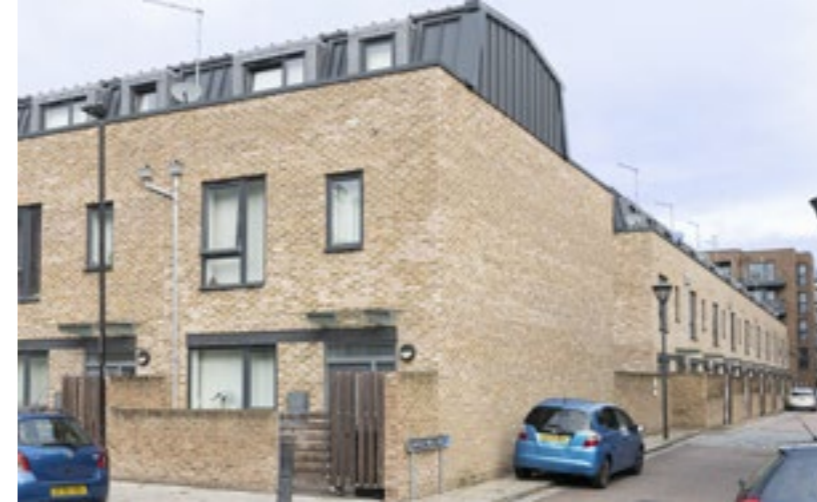
Edward Mills Way London (Tower Hamlets) Stockwool
