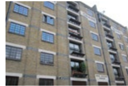
D. Grade II listed New Crane Wharf built in 1873 and reinstated in 1885 on Wapping High Street, within the Wapping Wall Conservation Area. It was converted into residential use and shops in 1990 and it is of stock brick.
