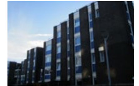
F. The post-war Lanfrac Estate, built as a result of clearance programmes. The estate is a uniform collection of blocks with up to 4 storeys. Some variation is added by the differing tone of the brick and the varying design of the plans.
