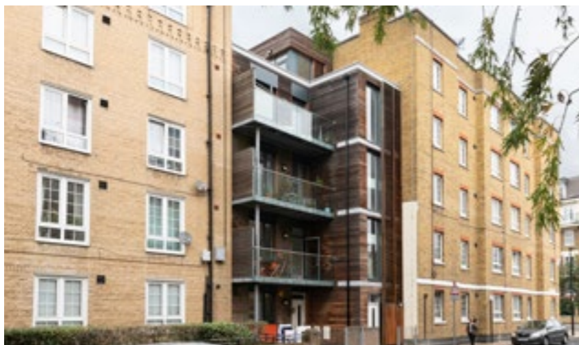
45 Prusom Street London (Tower Hamlets)
