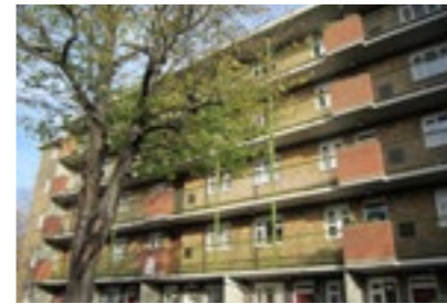
D. The post-war Park View Estate, from 1953, designed so as to allow views to Regent's Canal and Victoria Park. Within the Victoria Park Conservation Area, it is of brick with cantilevered balconies.
