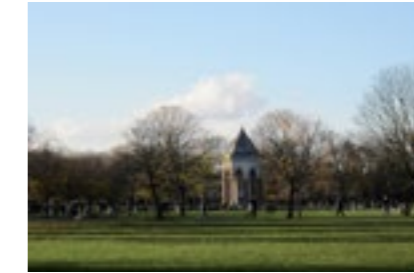
E. The Grade II* listed Baroness Burdett Coutts Drinking Fountain, also known as Victoria Fountain, built in 1862. It displays a Gothic-cum-Moorish style.
