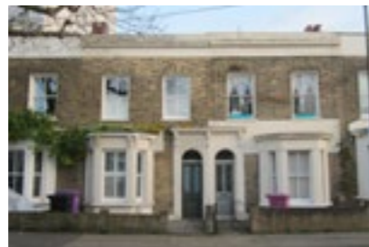
B. Late 1860s 2-storey terraces with canted bay window at ground floor and simple Victorian sash windows above, stuccoed details on ground floor, part of Swaton Road Conservation area.
