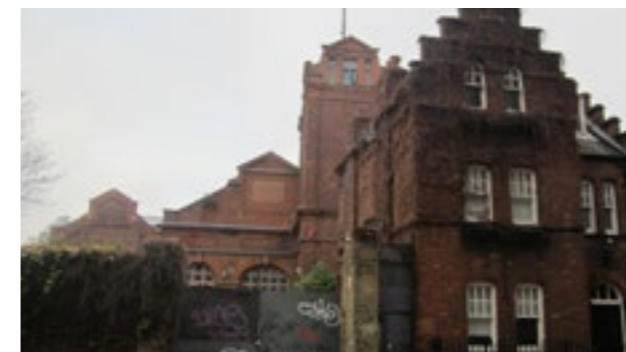
The Grade II* listed former Wapping Hydraulic Pumping Station from 1893, within the Wapping Wall Conservation Area.
