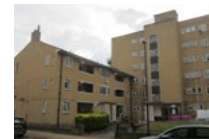
H. Mix of 3- and 6-storey blocks completed in 1951 and built with London stock brick and slate to reflect the existing housing stock of the area at the time, part of Lansbury Conservation Area.
