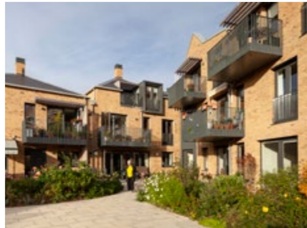
The Older Women's Co-Housing is a development of 25 self contained flats with shared communal facilities and gardens, managed on co-housing principles. (photo © Galit Seligmann & Pollard Thomas Edwards)
