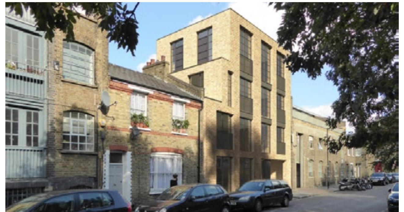
49 Derbyshire Street: The streetscape infill development (rendered image of approved scheme) implements materials that integrate well with surrounding buildings whilst mediating between the different heights and typologies. (image ©Rivington Street Studio)
