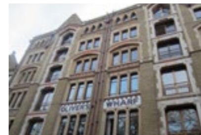
G. Grade II listed Oliver's Wharf built in 1880 on Wapping High Street, within the Wapping Pierhead Conservation Area, was Wapping's first warehouse to be converted into flats. It is of stock brick with red brick and stone dressings.
