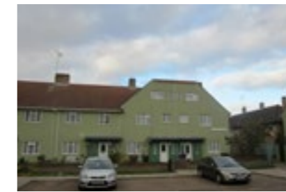
E. Limehouse Fields Estate, an original 1960s development with 2-3-storeys painted with stucco.
