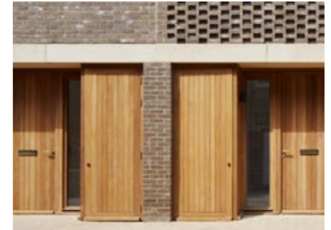
Bin and bike storage integrated into building design with recessed front door. (photo ©Jack Hobhouse & Morris+co)
