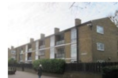
H. 3-storey post-war housing blocks built between 1957-1958 with plain brick panels, recessed private balconies and shallow gabled roofs.
