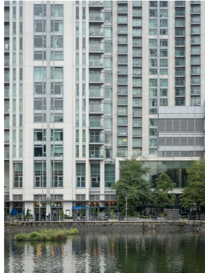
Full ceiling height windows are at risk of overheating in summer and heat loss in winter.
