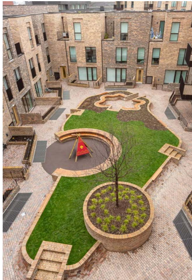
Terraces front onto communal amenity space.
