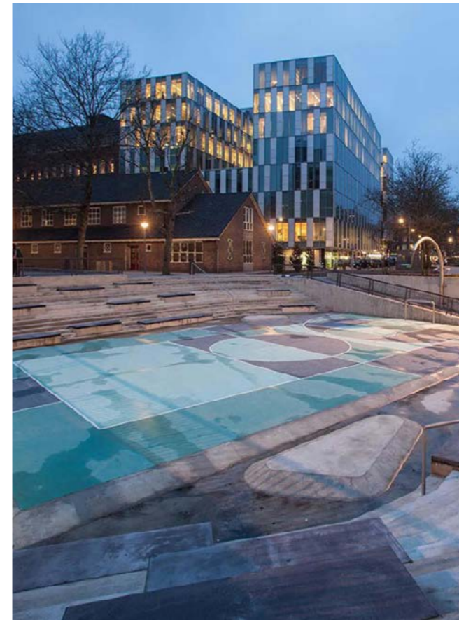
Public space incorporates a basketball, skateboarding features and seating but functions as flood water collection pools in storm conditions.
