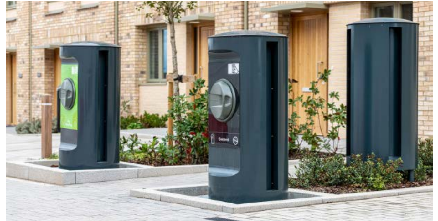
Envac System integrated into the public realm using similar material finishes.
