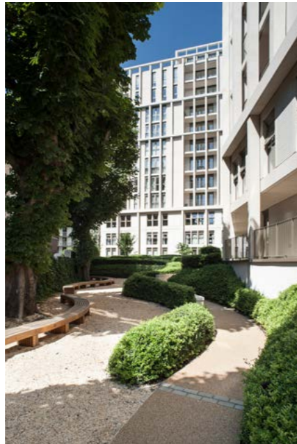
Abell and Cleland blocks, London, UK. DSDHA.
