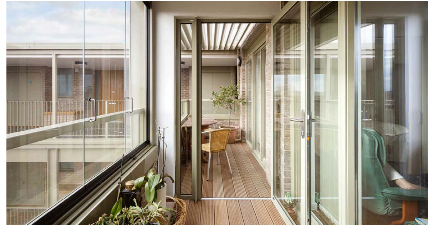
The environment of the wintergarden is easy to control by opening or closing large windows and doors.
