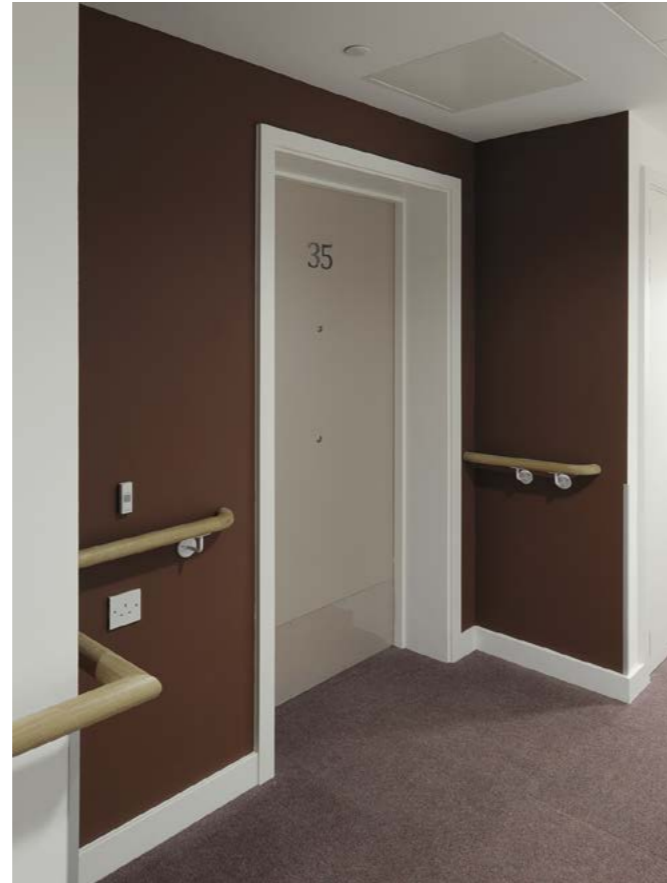
Door is staggered and colour provides personalisation and a sense of belonging.
