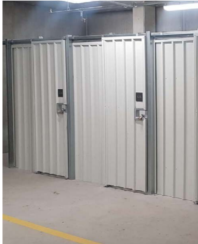
Secure basement storage lockers.
