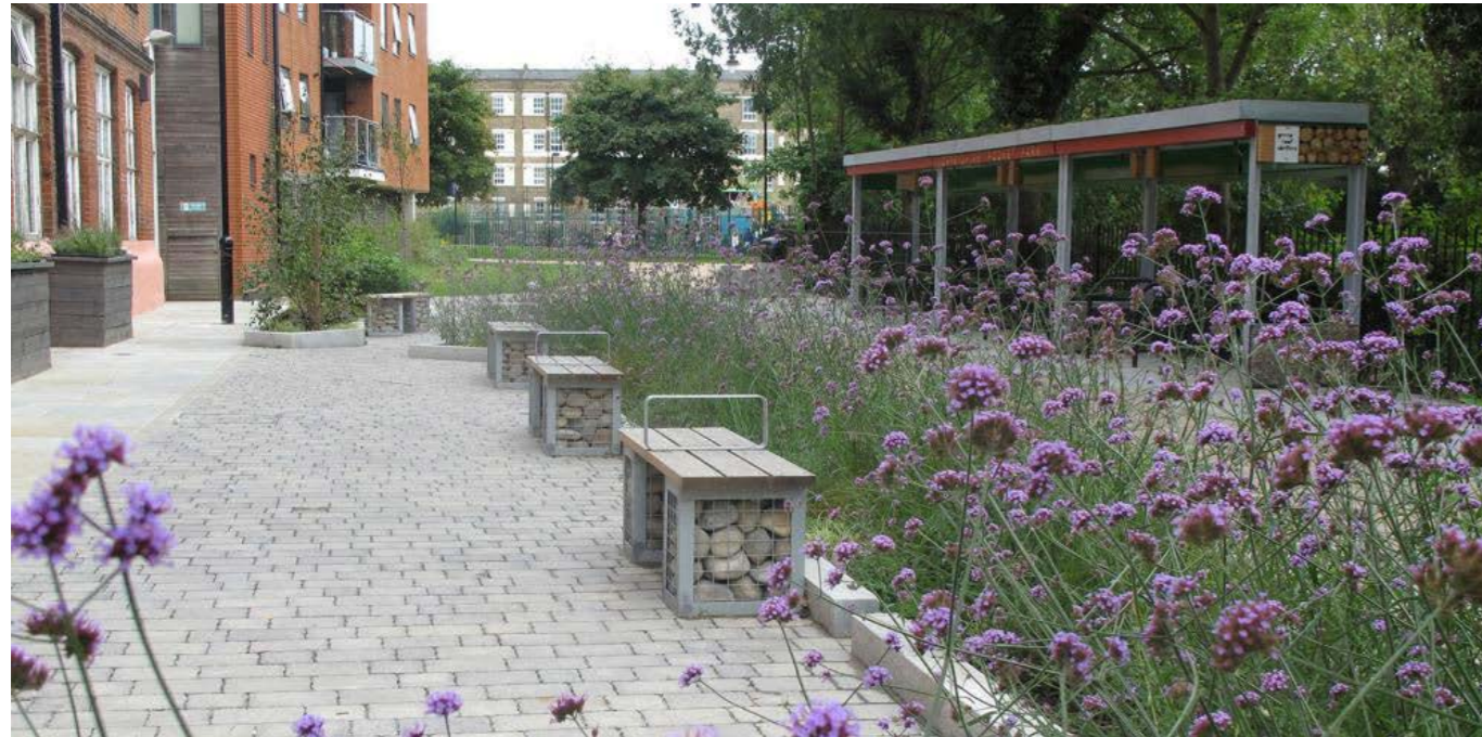
A range of sustainable drainage measures have been installed in Derbyshire Street pocket park, Tower Hamlets. These include green roofs, permeable paving, swales and rain gardens.
