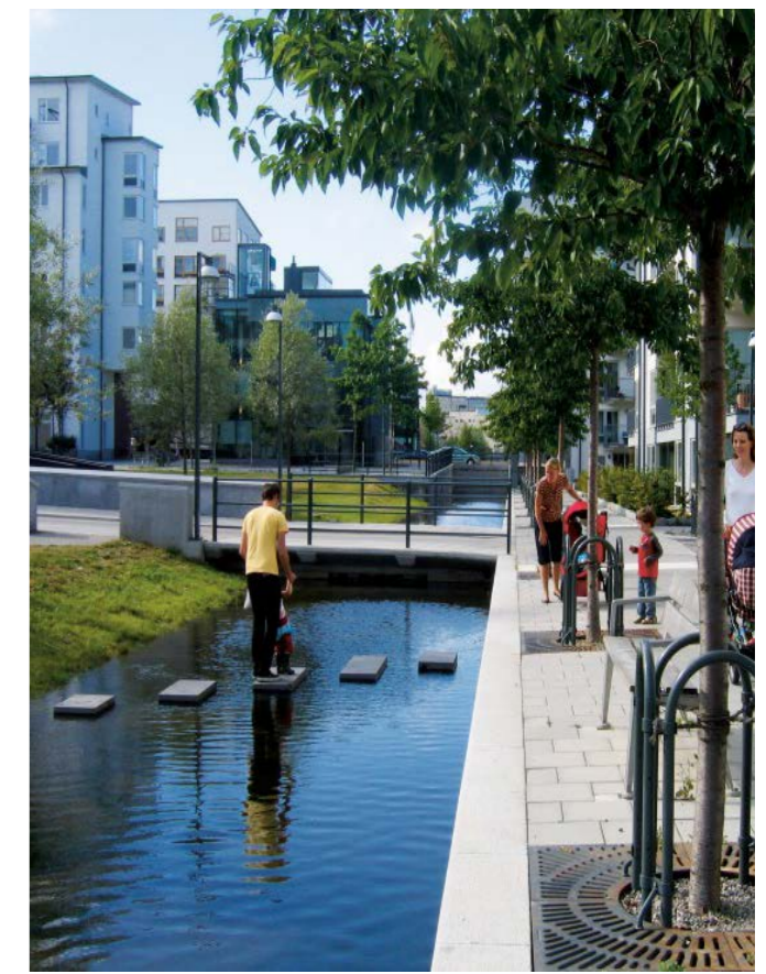
SUDs detention basin incorporated into public realm.
