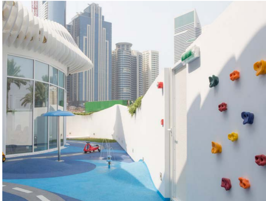
Childcare outdoor play space is located on a terrace but design provides privacy and safety.
