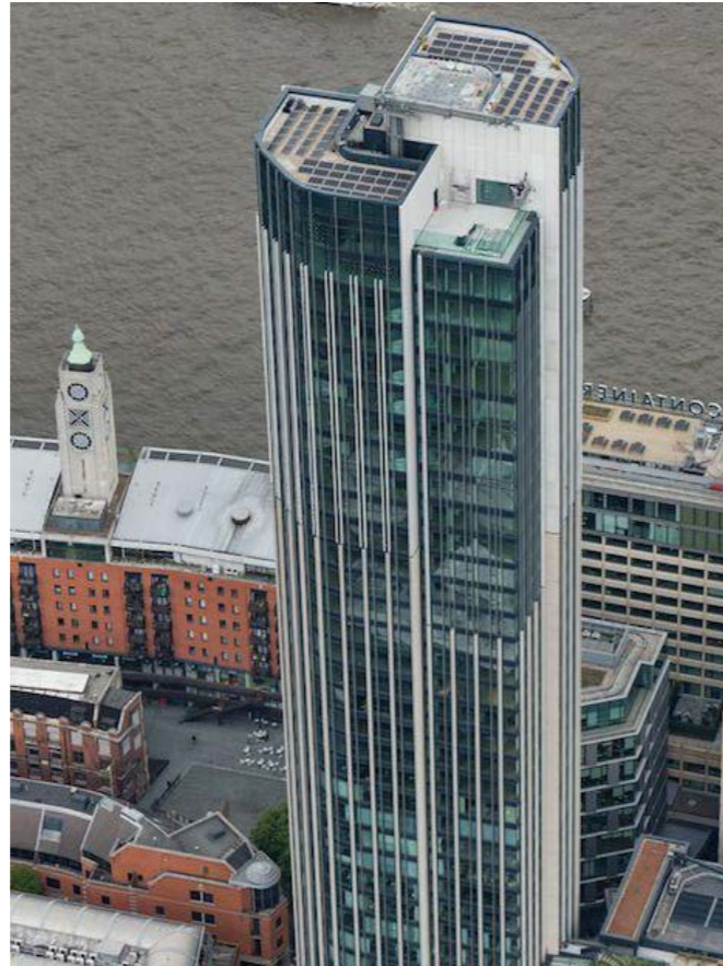
Solar panels are integrated into the design of the building, located on the roof and the cladding of the top floors.
