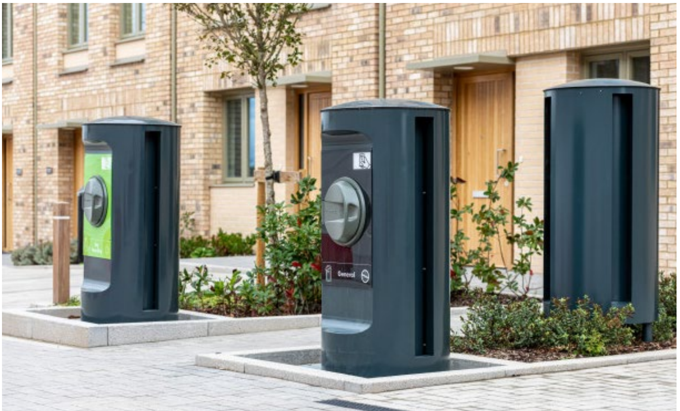
Fig. 6. Automated Waste Collection System intake hatches within the public realm.
