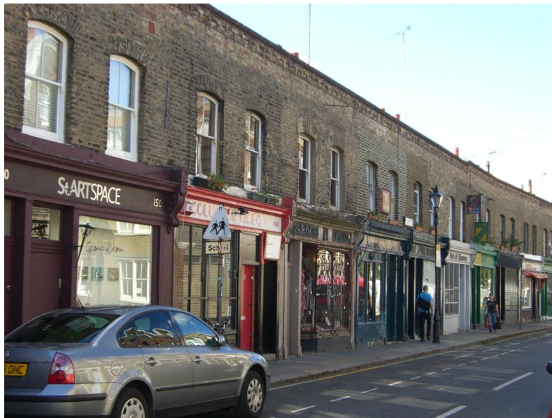
London (or Butterfly) roof - street elevations in Wimbold Street and Columbia Road (above): This type of roof, concealed from the street behind a continuous parapet is highly characteristic of large parts of the Jesus Hospital Conservation Area. This consistency is important to the character and appearance of the conservation area.
