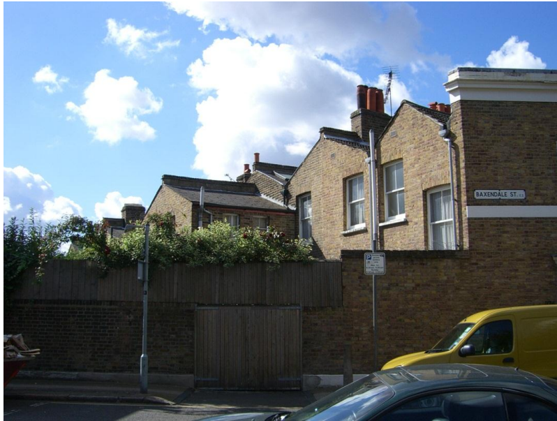
London (or Butterfly) roof (above): rear elevation of Barnet Grove from Baxendale Street. The parapet is omitted from the rear elevation of houses with London roofs, exposing the distinctive pattern of gables and valleys to view.
