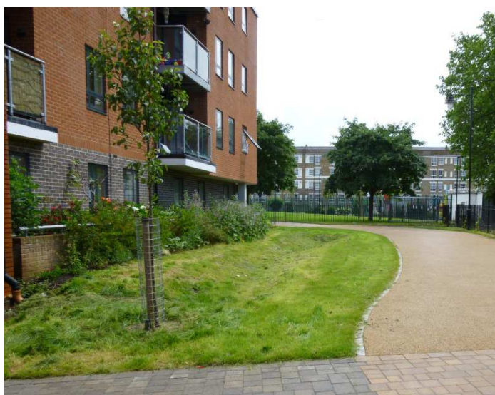
Figure 2.11 Swale, Derbyshire Street, Tower Hamlets
