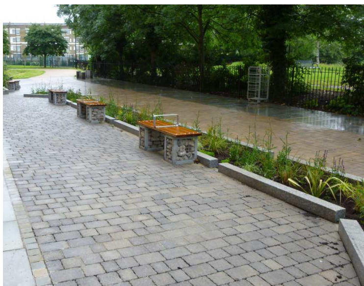
Figure 2.13 Permeable Paving Derbyshire Street, Tower Hamlets
