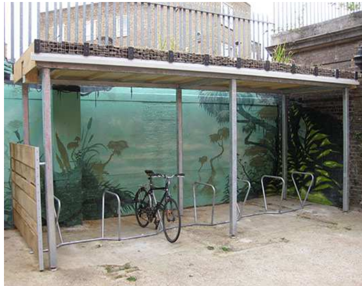
Figure 2.8 Green roof application on a bike shelter ©Green Roof Shelters
