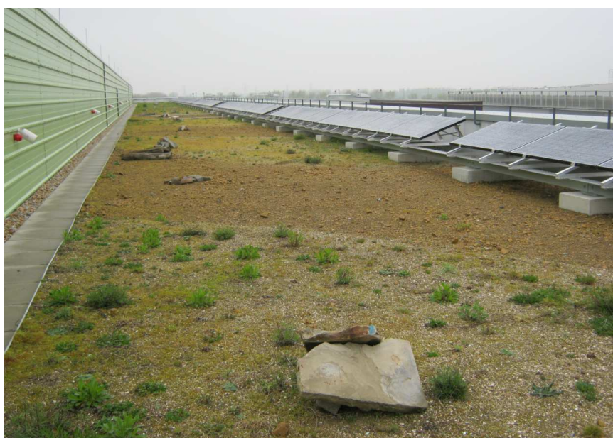
Figure 2.6 green roof at the Queen Elizabeth Olympic Park © University of East London
