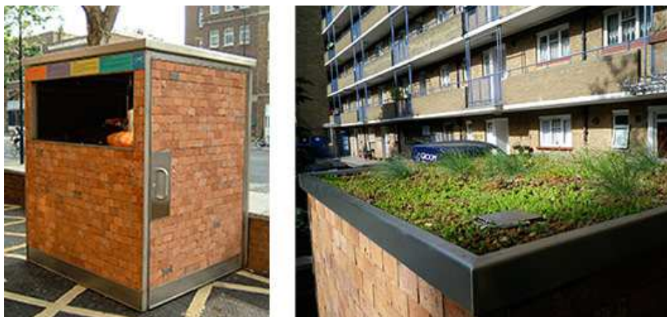
Figure 2.9 Pre-fabricated Green roof bin store ©Green Roof Shelters
