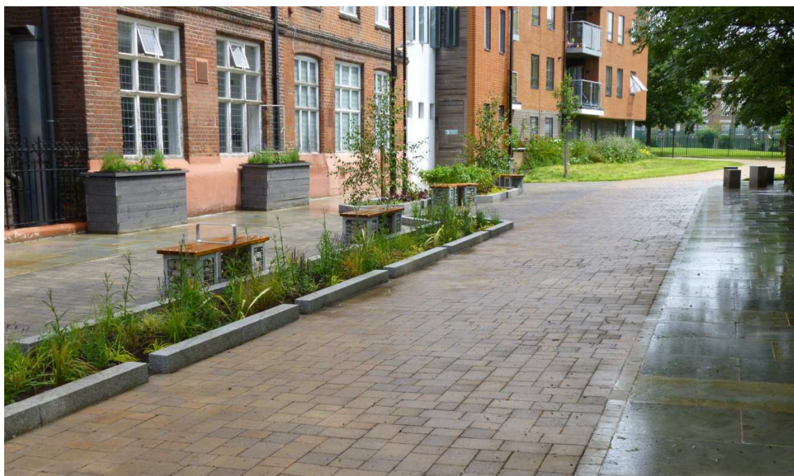
Figure 2.2 Rain Garden, Derbyshire Street, Tower Hamlets
