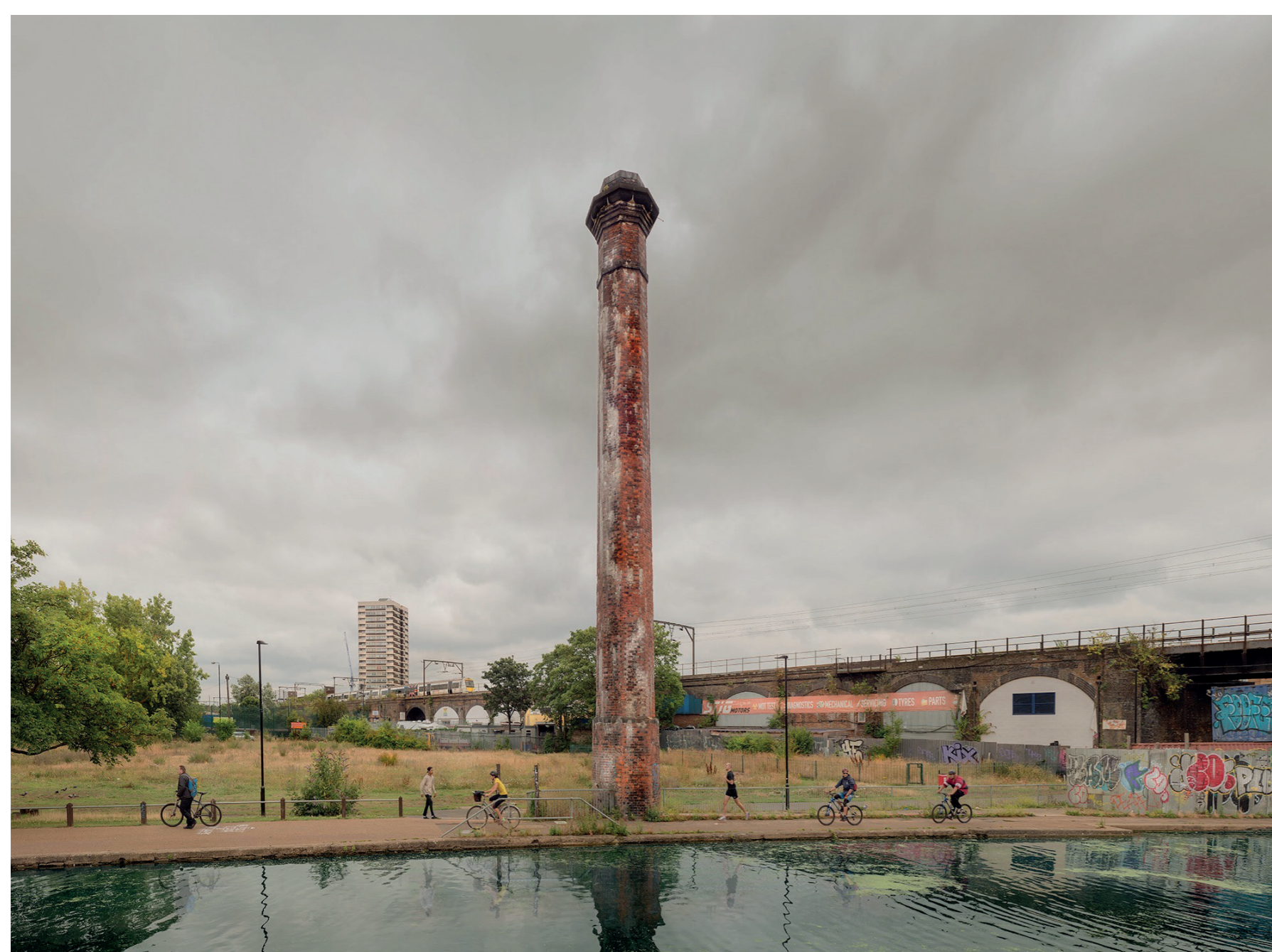
Victorian Chimney beside Regents Canal
