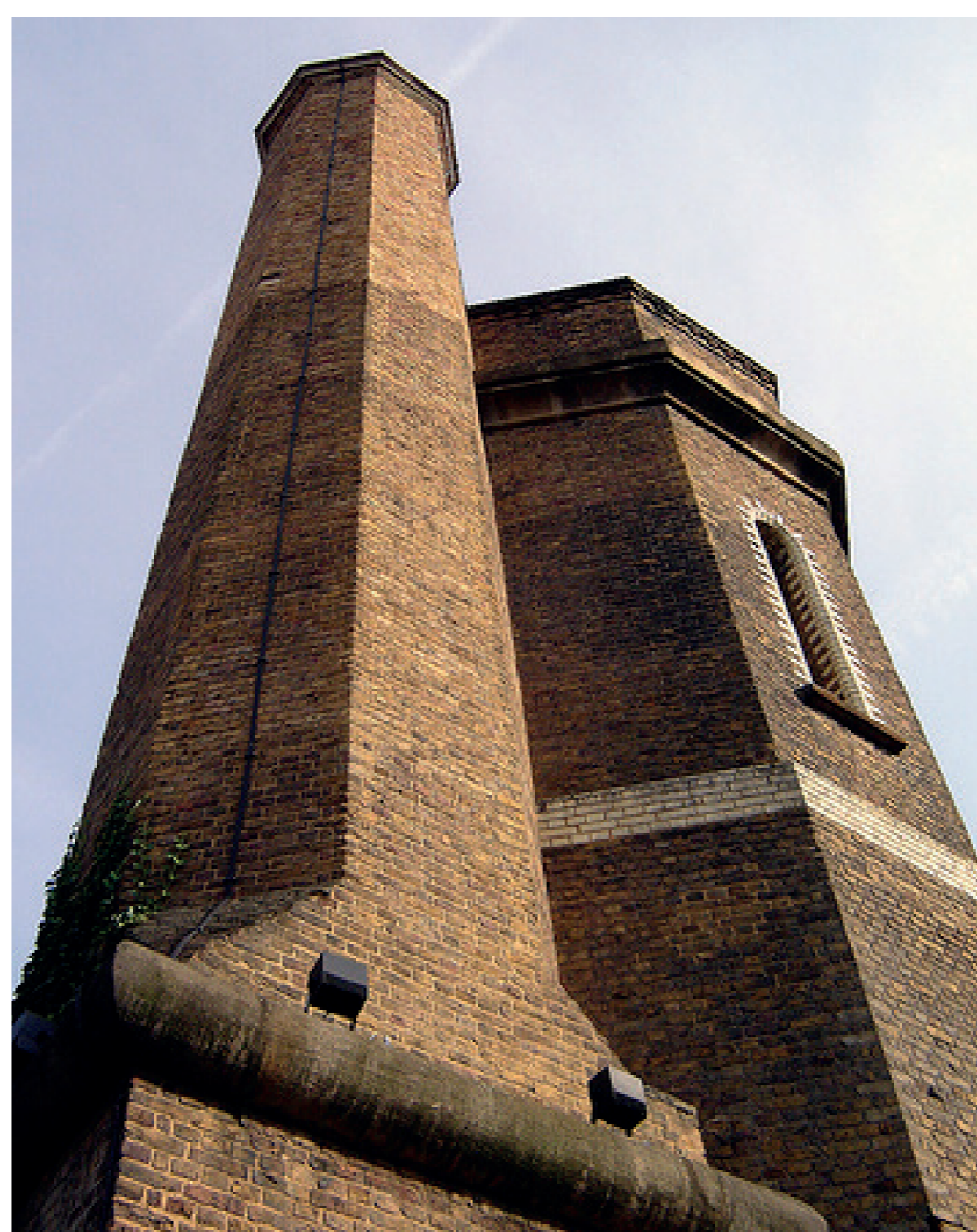
Accumulator tower at Limehouse Cut
