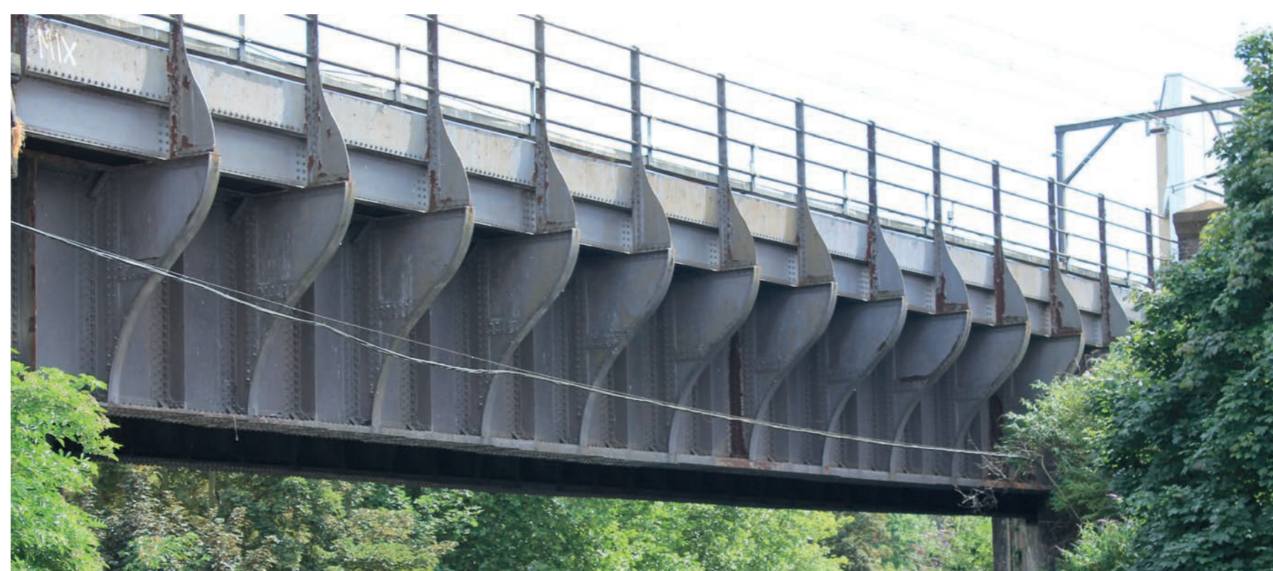
Adjacent Railway Bridge
