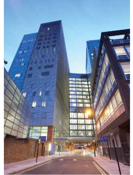
Entrance to new RLH building on Stepney Way
