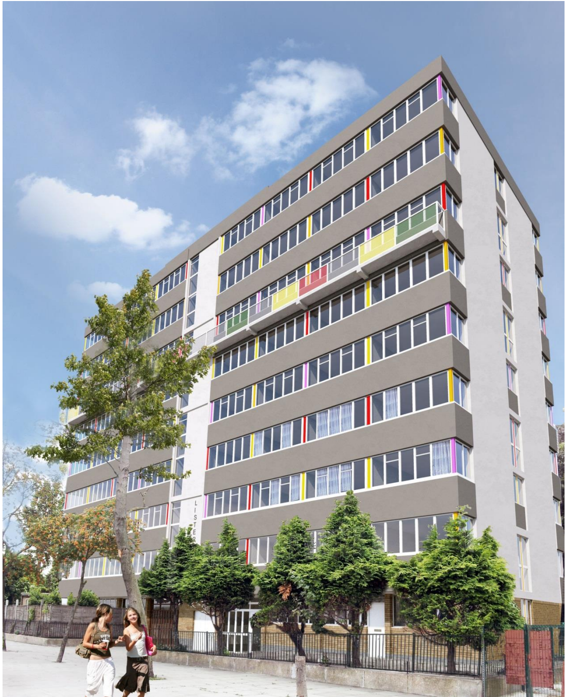
Picture 3 – Visualisation of Lister House, following EWI works
