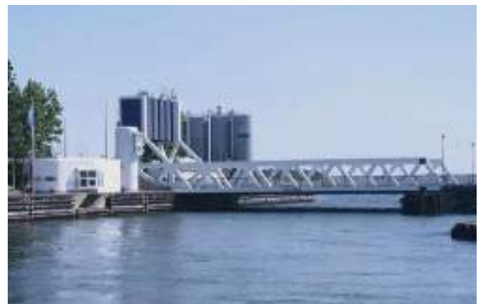
Modern rolling bascule bridge
