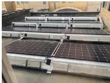
It is projected that the project will reduce the electricity demand of the office by 2,638 kWh a year which is a carbon emission reduction of 1.5tCO2.
