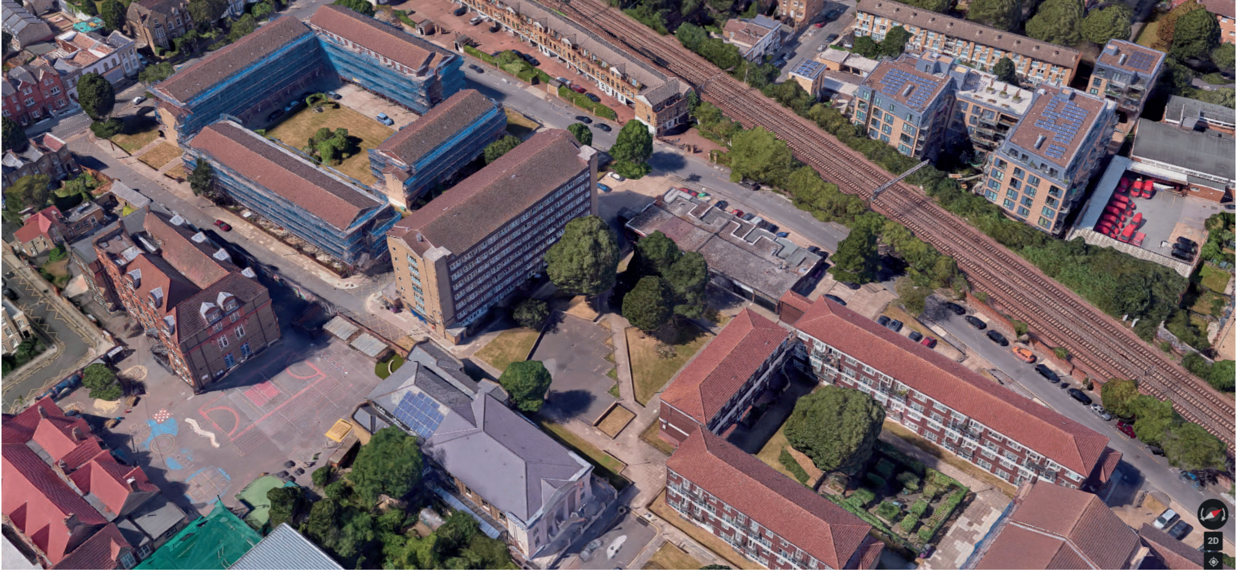
EXISTING AERIAL VIEW OF SITE
