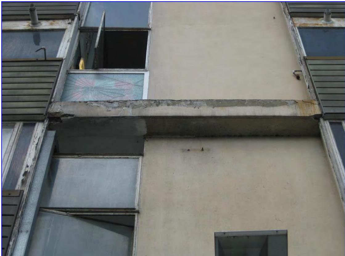
Photograph 12: Closer view of the 3<sup>rd</sup> floor slab edge over the entrance with spall to the left apparent as well as deteriorated coatings. Note also broken glazing and poor condition timberwork.
