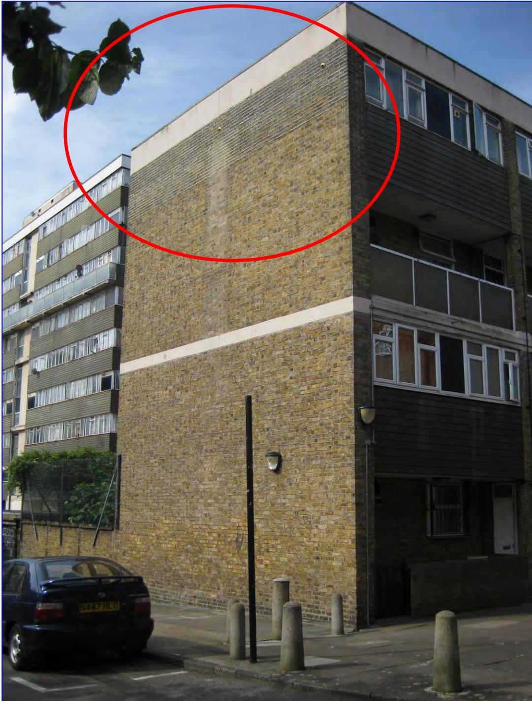
Photograph 14: General view of east gable to Treves with repointed top section of brickwork apparent.
