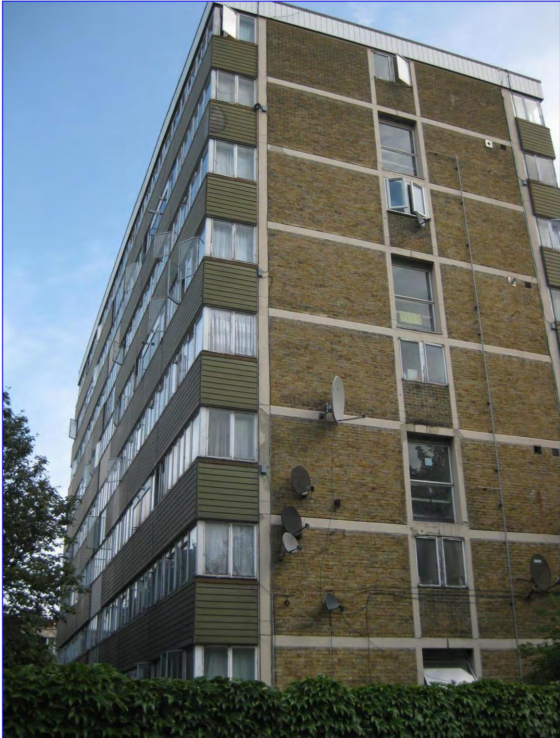
Photograph 3: General view of Lister House, main west elevation and south gable. Note the exposed concrete frame to the gable as well as brickwork wall panels.
