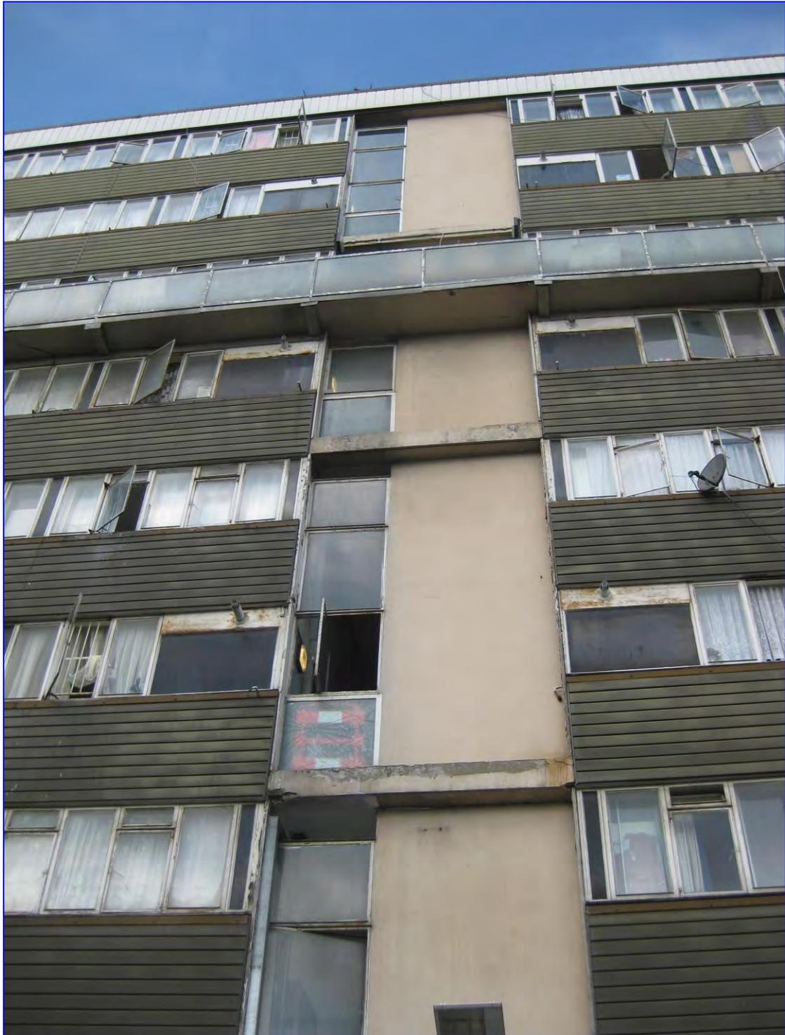
Photograph 2: General view of the central (stair/lift/bin chute) section to the east elevation, with exposed floor beams at alternate floors and an access walkway at 6<sup>th</sup> floor. The rest of the elevation is clad.
