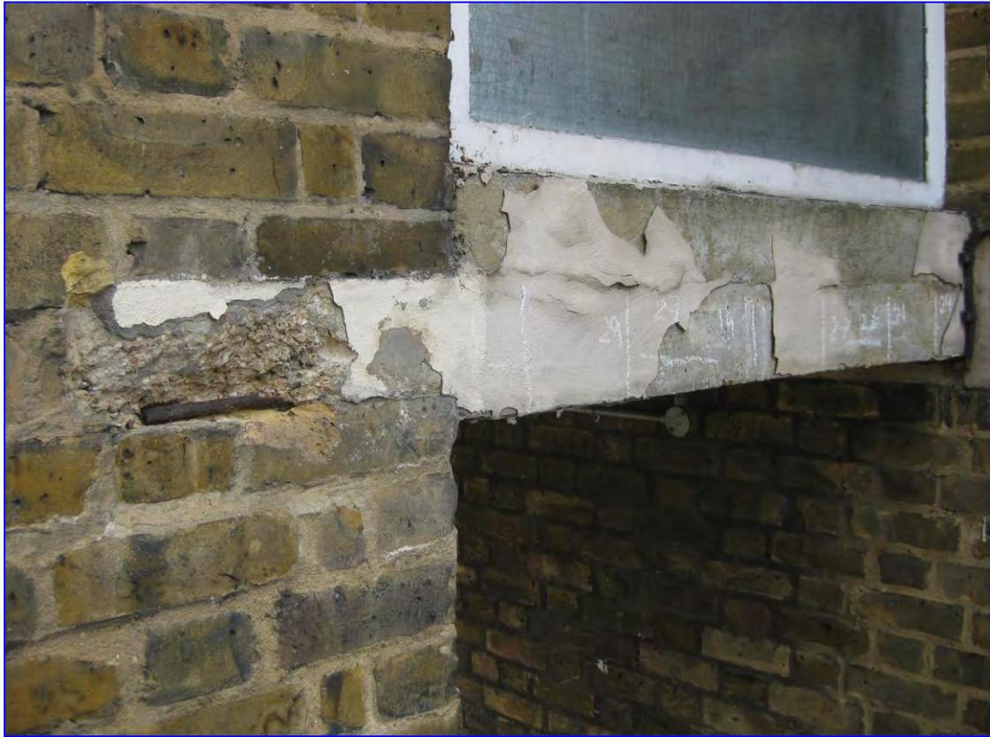
Photograph 15: Example of deteriorated coatings and a spall to concrete in access stairs.
