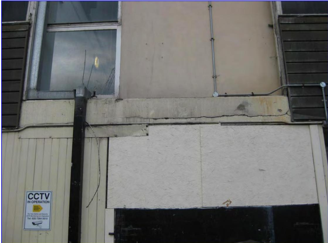
Photograph 11: Closer view of the first floor cracked slab edge, Lister House.
