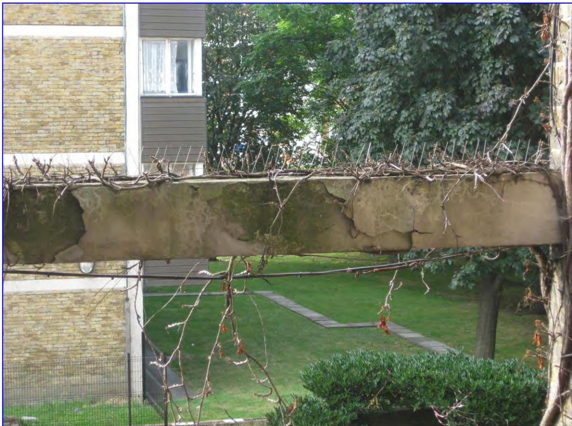
Photograph 16: Example of further deteriorated coatings to a flying beam in the access area. Note also plant growth.
