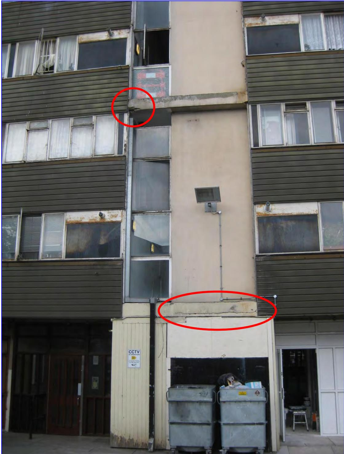
Photograph 10: General view at the main entrance to Lister House with spalling/cracked concrete indicated.
