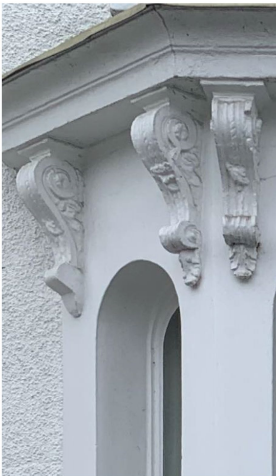
Stucco console brackets
