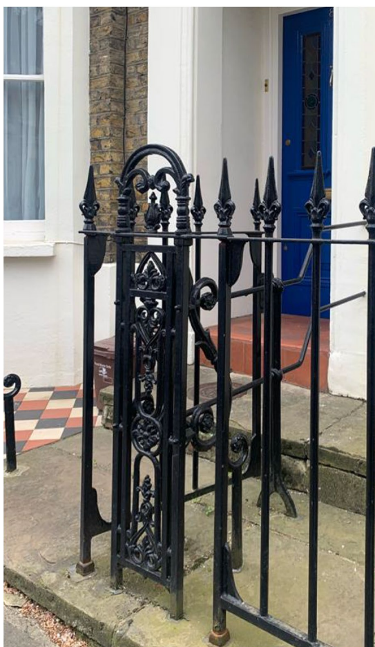
Cast iron railings
