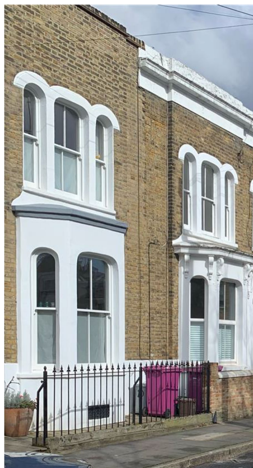
Cast iron railings
