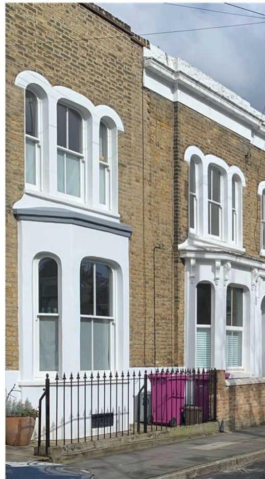
Cast iron railings
