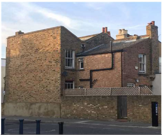
Corner property with inboard staircase
