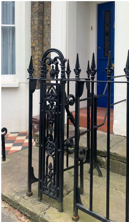
Cast iron railings
