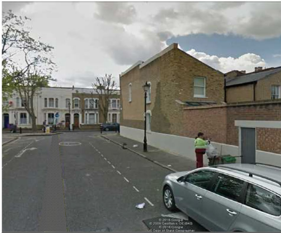
Corner property with outboard staircase
