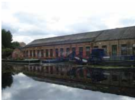
Former Screw Stopper Factory
