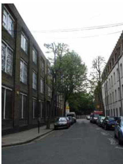
View towards eastern end of Dace Road
