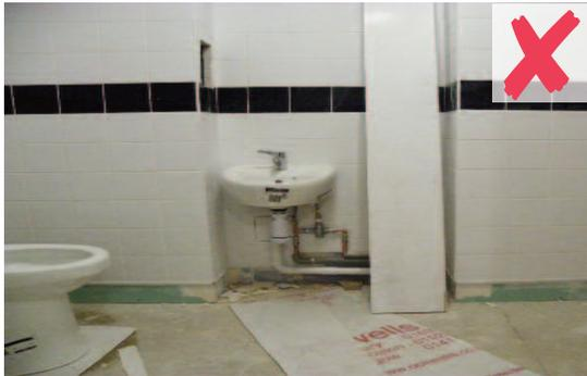
Image on the left: bathroom in new development on Old Bethnal Green Road. Spacious and well detailed apart from sink which the manufacturer claims is DDA compliant it is not.
