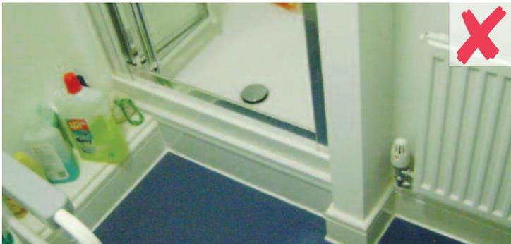
The same bathroom showing the tortuous access into the shower. Best practice could have floor drainage/wet room to enable step free access.
