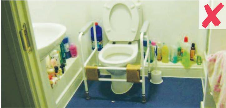
The bathroom walls are not robust enough to take grab rails – which have prevented drop down rails being fitted, resulting in bulky free standing frame round toilet further reducing manoeuvring space
