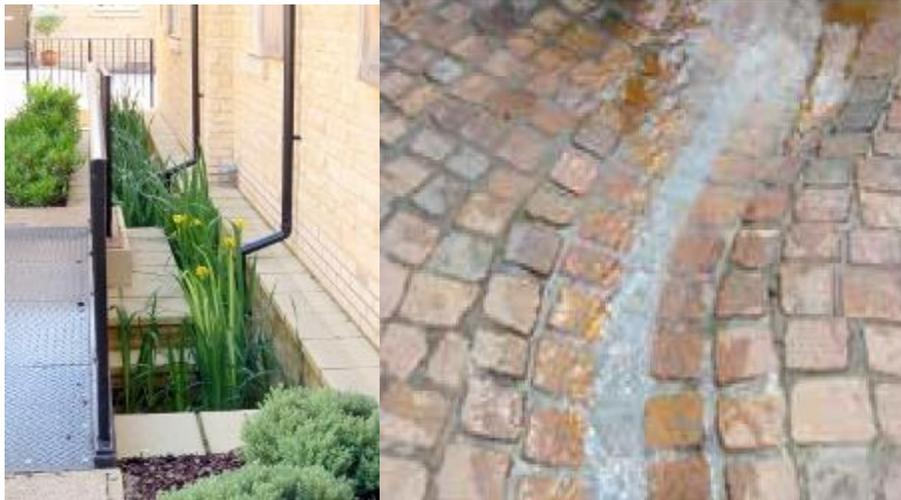
Figure 6-8 Example of drainage channels and rills. SuDS Manual C753.
