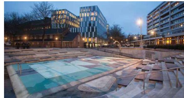
**Figure 6-21 Example of urban hard surfaced off-line detention basin. SuDS Manual C753.**
