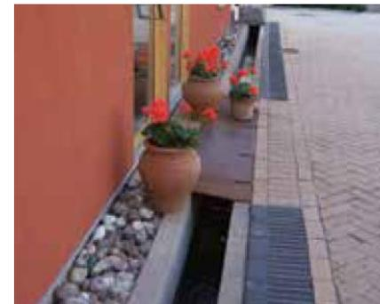
**Figure 6-12 Example of rills that convey runoff along the surface. SuDS Manual C753.**
