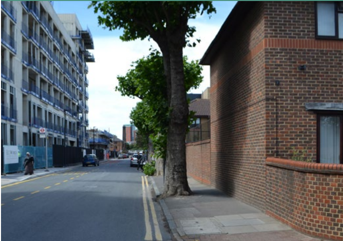
↑ Mature trees' pits clash with footpath on Blair Street restricting footways and causing uneven surface
