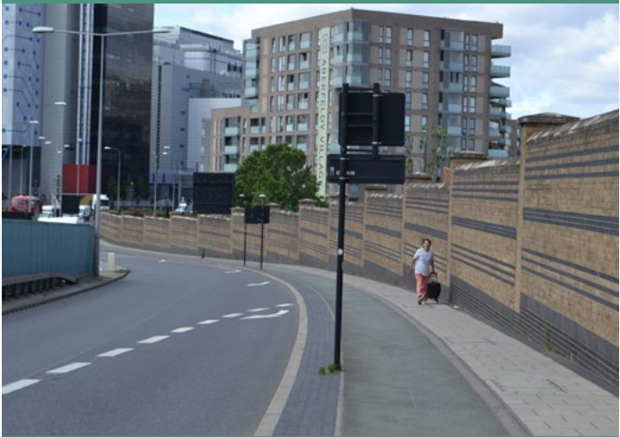
↑ Walled footpath on A13 is signed as shared use but is low quality and narrow
