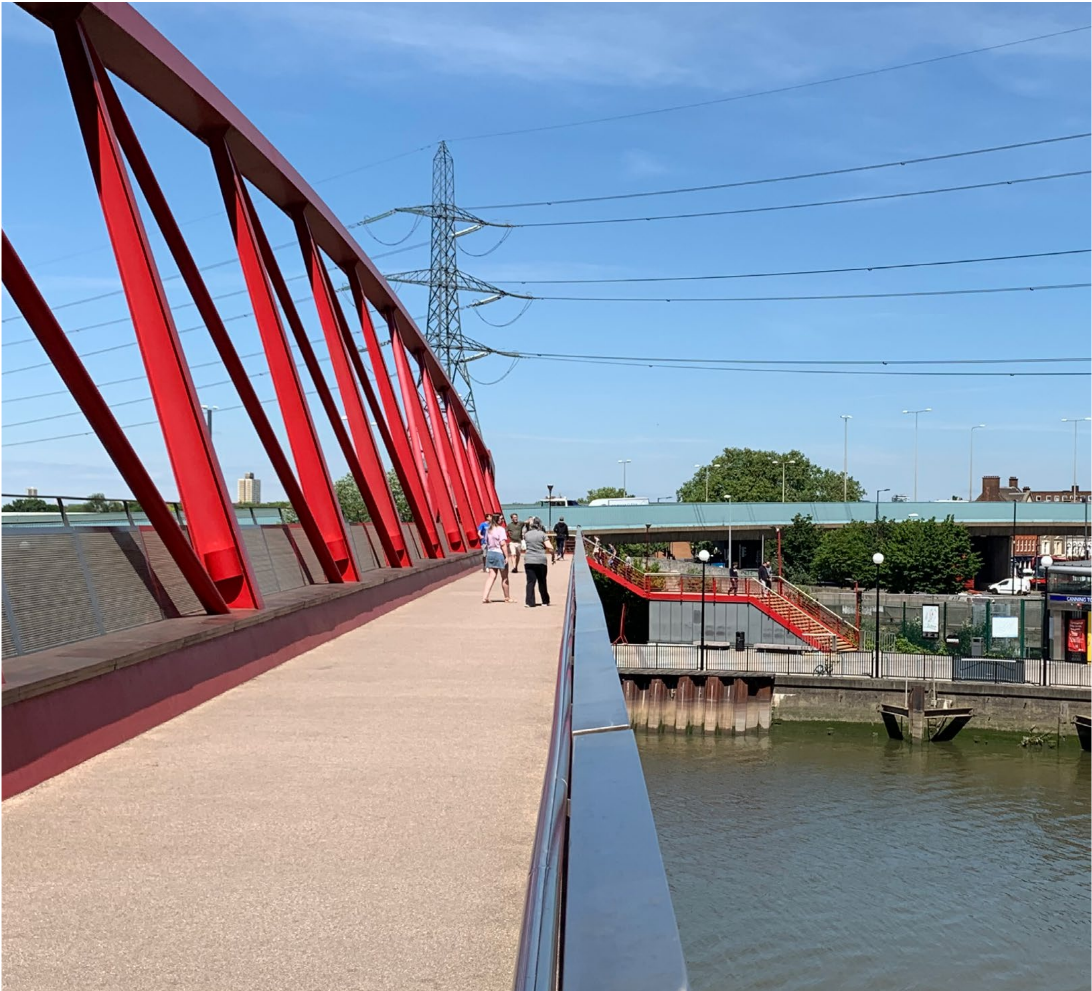
› The ‘Red Bridge’ built with developer contributions relating to the City Island development and crossing Bow Creek at the mouth of the River Lea. The bridge is able to rise by 4m on pneumatic pistons in the event that a taller ship requires access up the River Lea beyond this point
