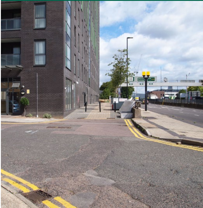
↑ Slip road from A12 to Teviot Street near Tweed Walk is excessively wide and encourages high vehicle speeds creating hostile pedestrian environment
