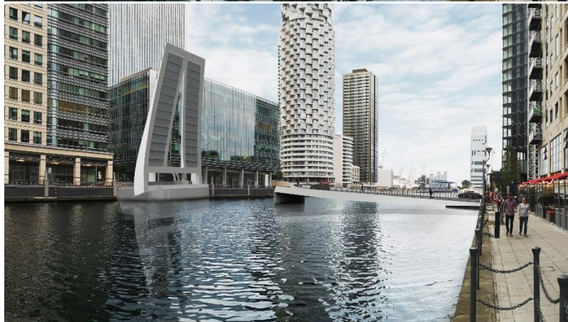
Figure 3.1 - South Dock Bridge – Isle of Dogs
