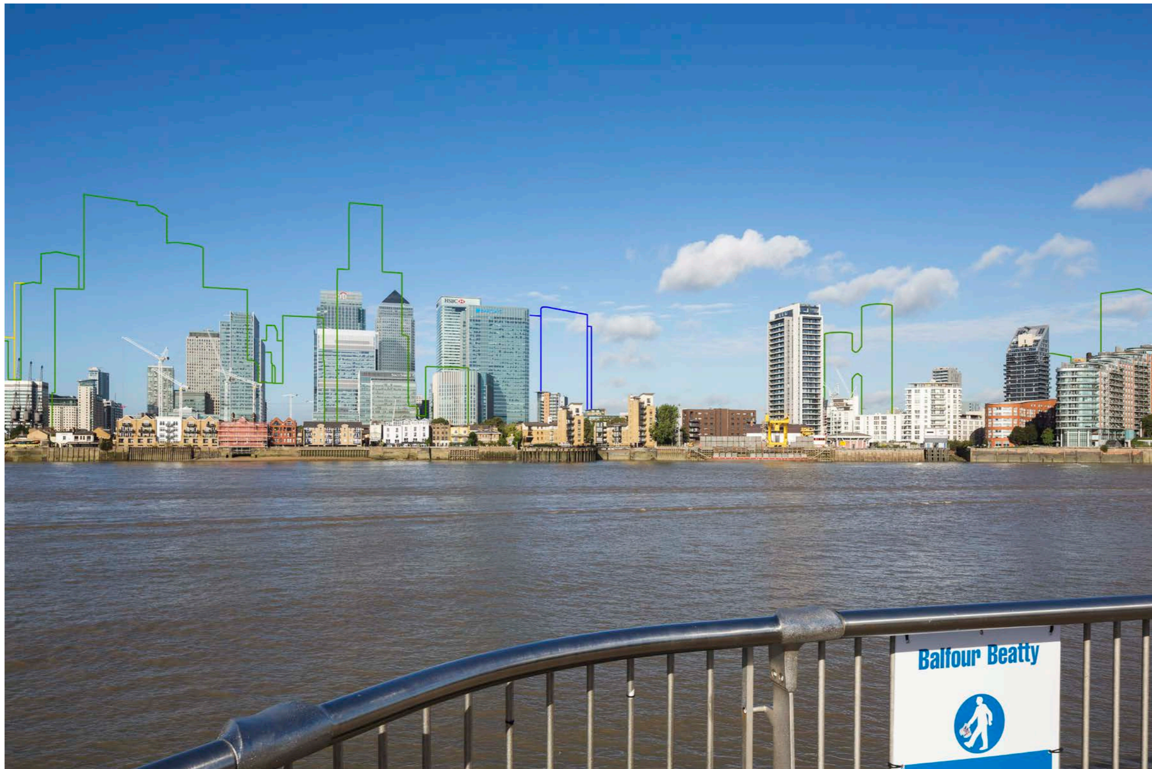
Figure 5a. View from the Greenwich peninsula (west of Canary Wharf) showing of Canary Wharf cluster and schemes with planning consent.
