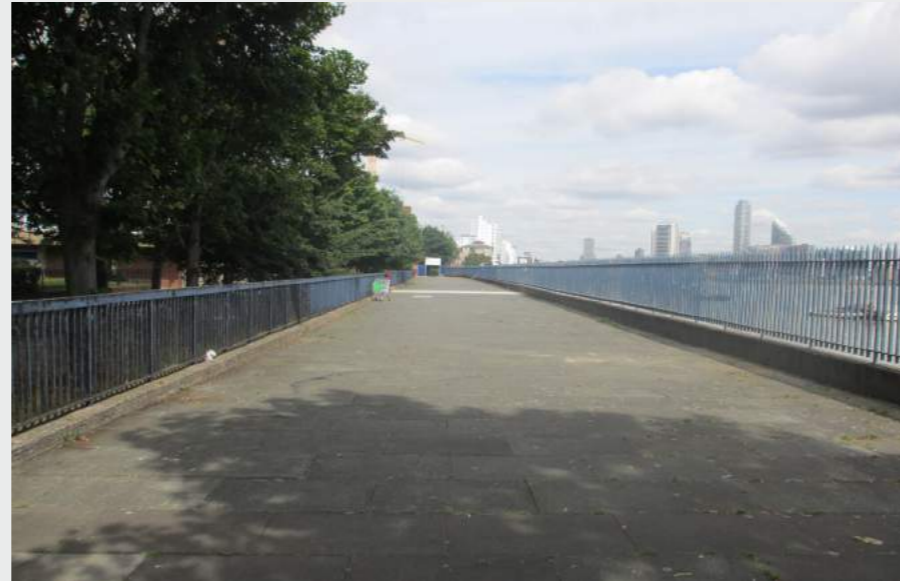
Empty pathway with barriers.
