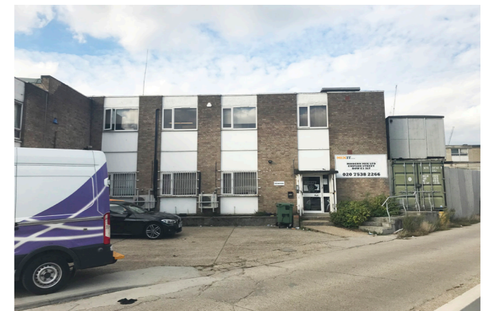
24 Building 19 - Mixit Concrete
