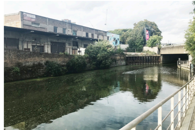
31 Limehouse Cut - South Boundary to Buildings 21 & 22
