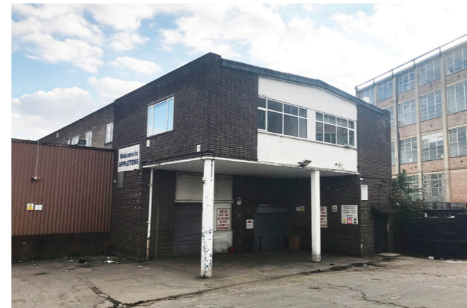
32 Building 23 - Appleton Warehouse - Office block
