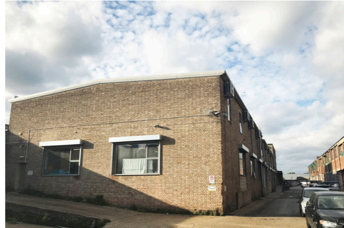
4 Building 3. Brickfield Studios. From South East
