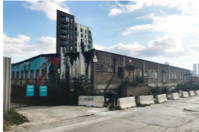
28 Building 22 - From North East
