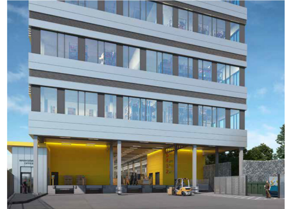
Loading docks, accessed from the car park & yard, accommodating HGVs.
