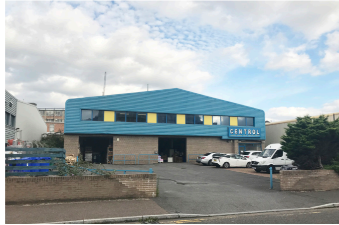
16 Empson Street West - St Andrews Way - West
