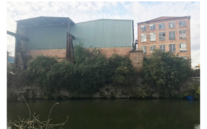
35 Limehouse Cut - South Boundary to Buildings 2 & 13
