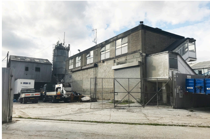
25 Building 20 - Mixit Concrete
