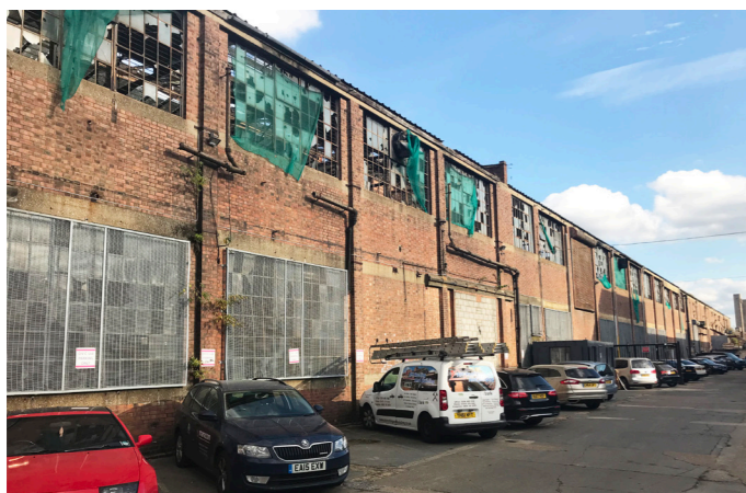
3 Building 2 - John Stevenson & Sons. Vacant. From North West
