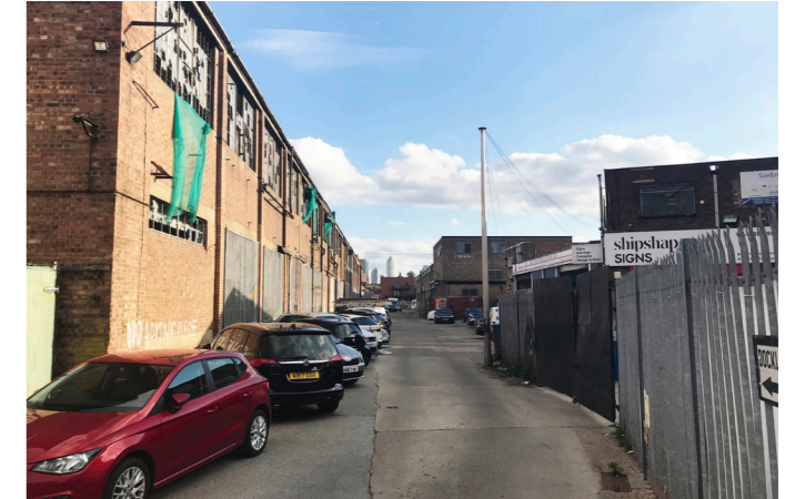
10 Brickfield Road from North
