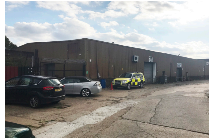
31 Building 23 - Appleton warehouse - From North East
