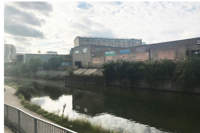
32 Limehouse Cut - South Boundary to Buildings 23& 13
