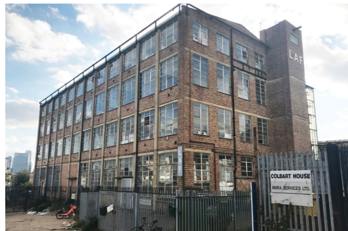
18 Building 13 - Old Hackney College. Limehouse Arts Foundation
