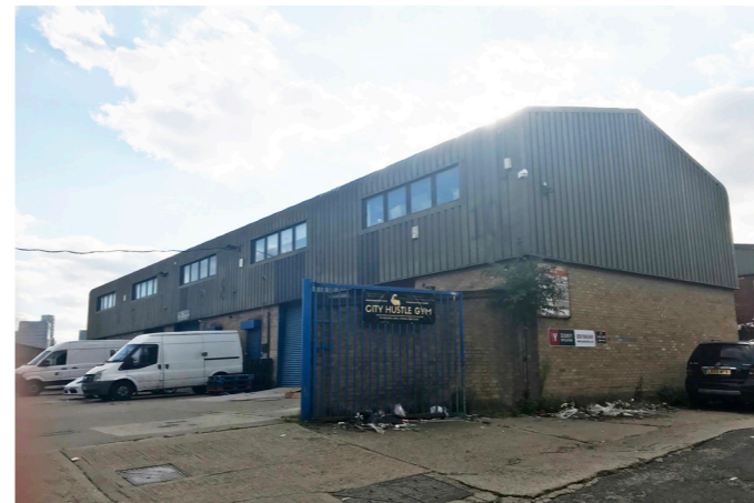
20 Building 16 - From North East
