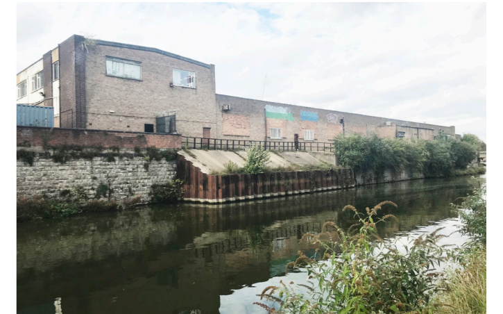
34 Limehouse Cut - South Boundary to Building 23
