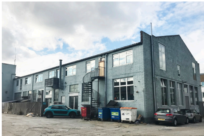
14 Building 9 - From South East
