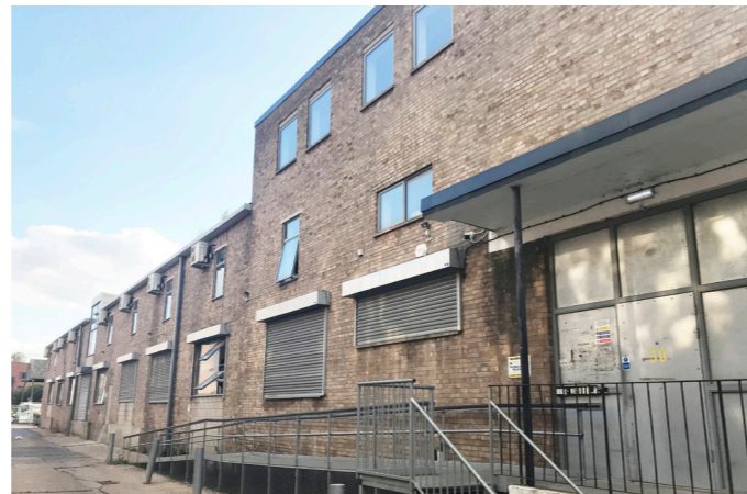
5 Building 3. Brickfield Studios. From North East
