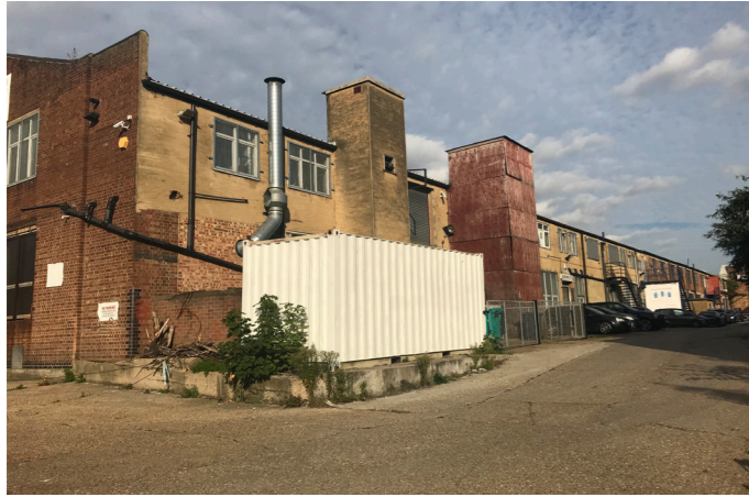
13 Building 9 - London Lifestyle Interiors. From South West.
