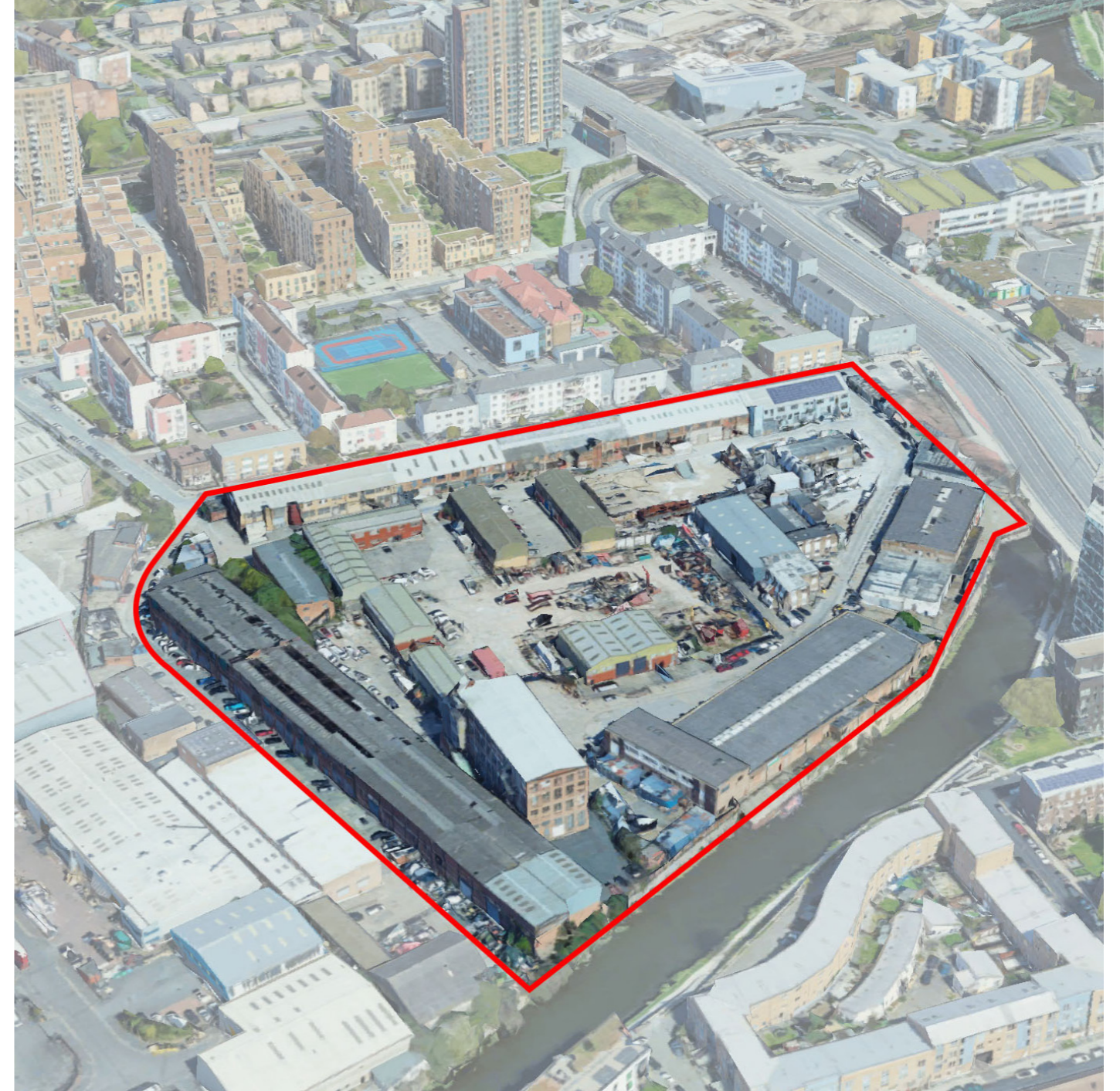
View toward North East
