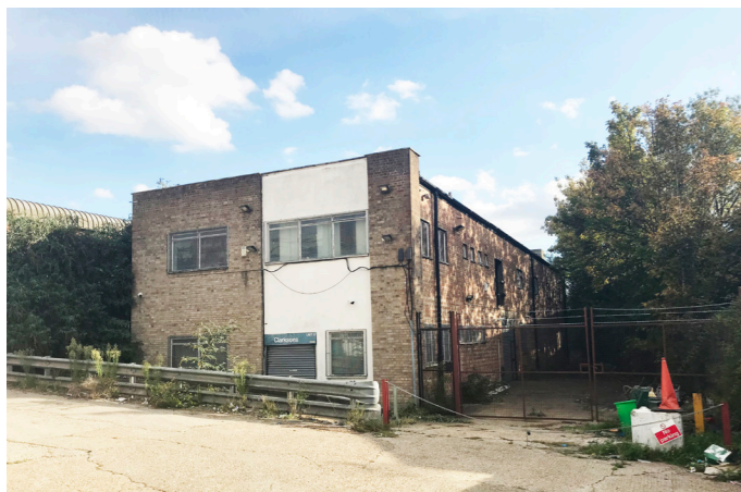
15 Building 10 - YY Security Installations
