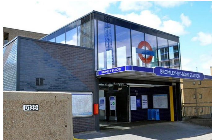
1 Refurbished Bromley By Bow Tube Station - A12
