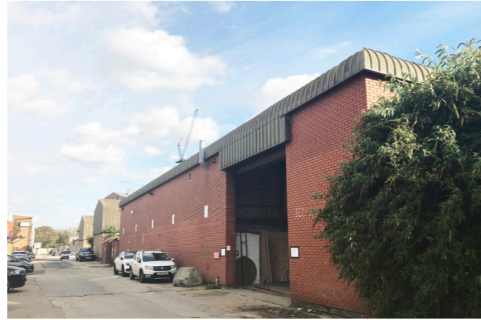
16 Building 11 - From North East
