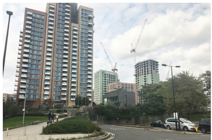
3 Twelvetees Crescent - A12 Under-pass
