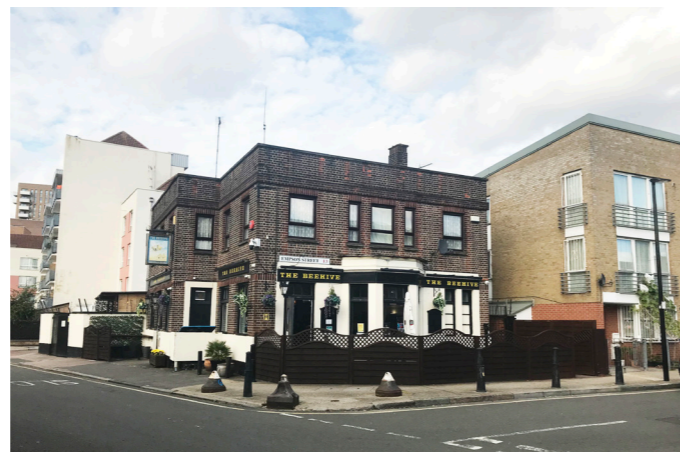
18 Empson Street Corner - The Beehive Public House
