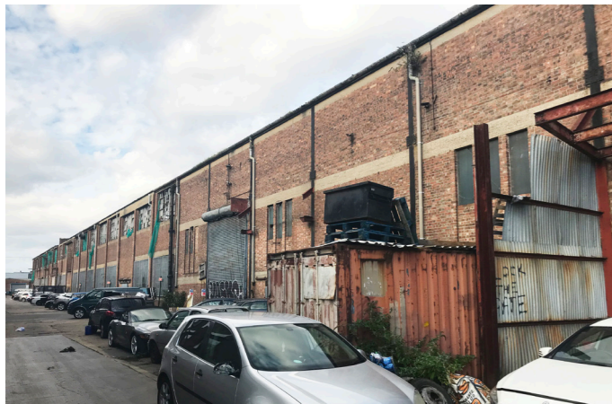
2 Building 2 - John Stevenson & Sons. Vacant. From South West
