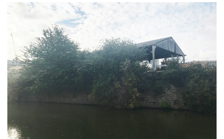
36 Limehouse Cut - South Boundary to Buildings 1
