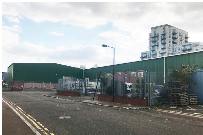
15 Empson Street West - St Andrews Way - West
