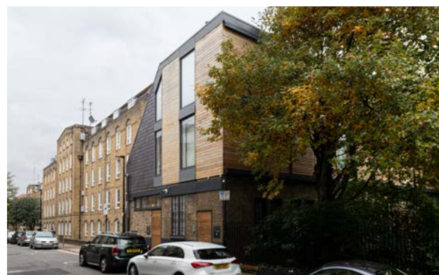
Slate wall tiles and timber cladding respond well to surrounding industrial character and brick façades. Good detailing have ensured that the cladding materials have weathered well. (photo ©Ivan Jones)
