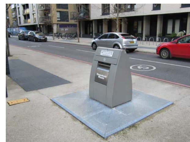
Example of Underground Refuse Stores.
