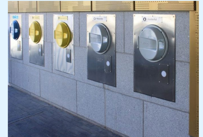
Fig. 14. An example of an AWCS portal area, demonstrating ease of access. Image courtesy of Envac.
