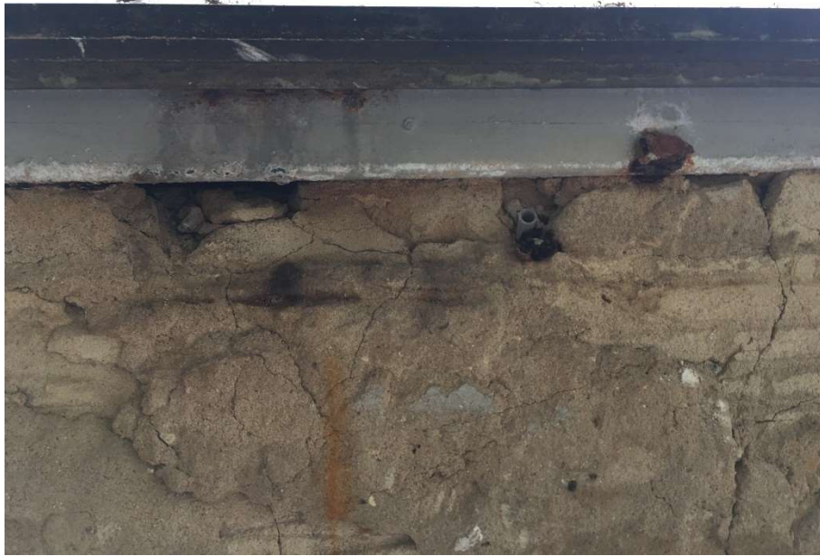
Close up view of wall window interface
