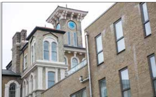
(12) Old and new, side by side at St Clement’s
