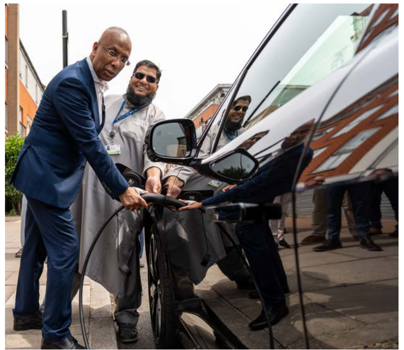
The charge points are being installed in existing lampposts
