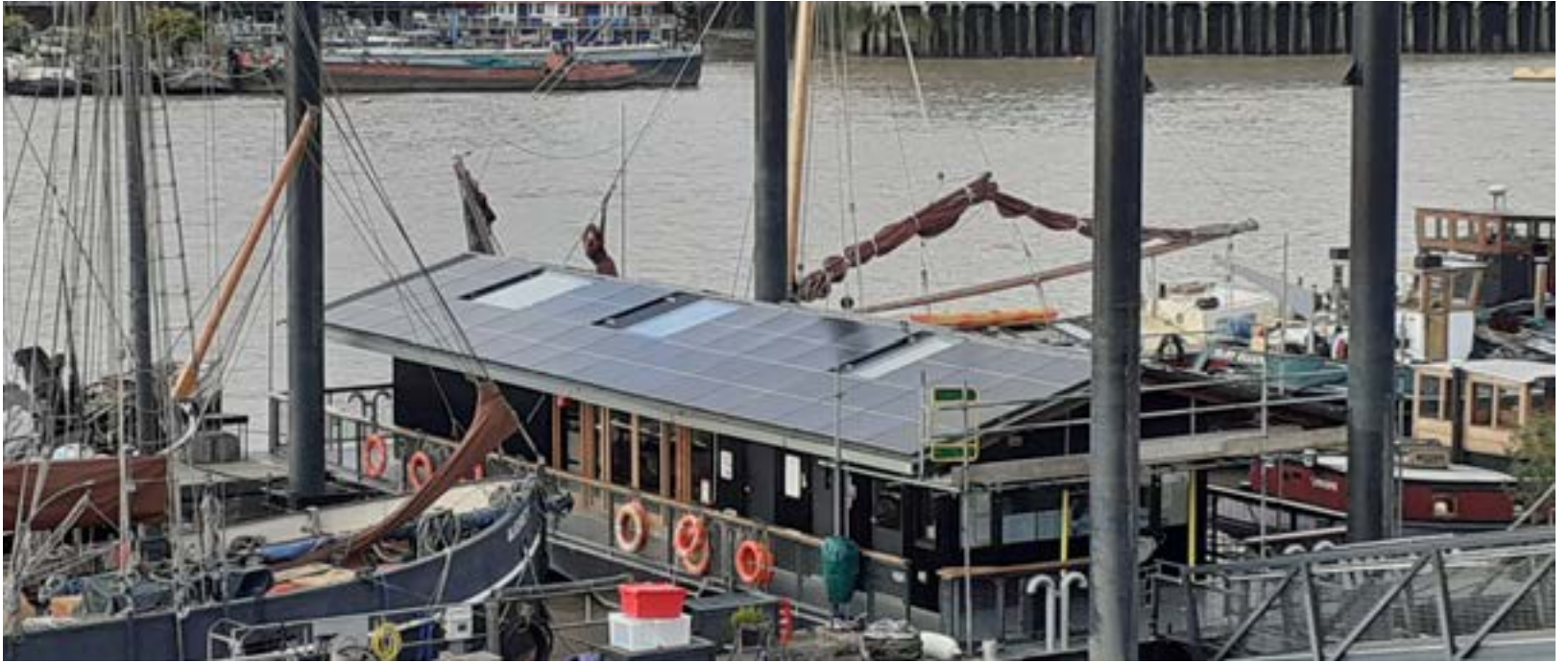
The Heritage Community Moorings with the solar panels funded by the grants programme
